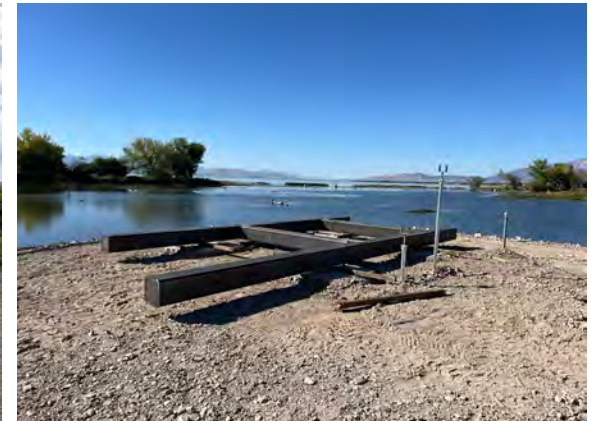
Metal base at wildlife viewing tower site
