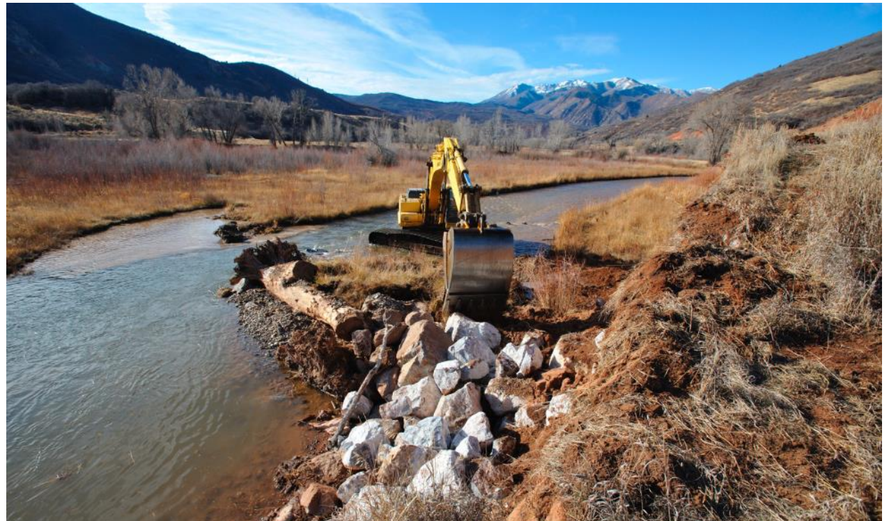
Aquatic and Riverine Restoration Construction, Diamond Fork River. Photo Courtesy Tyler Allred
