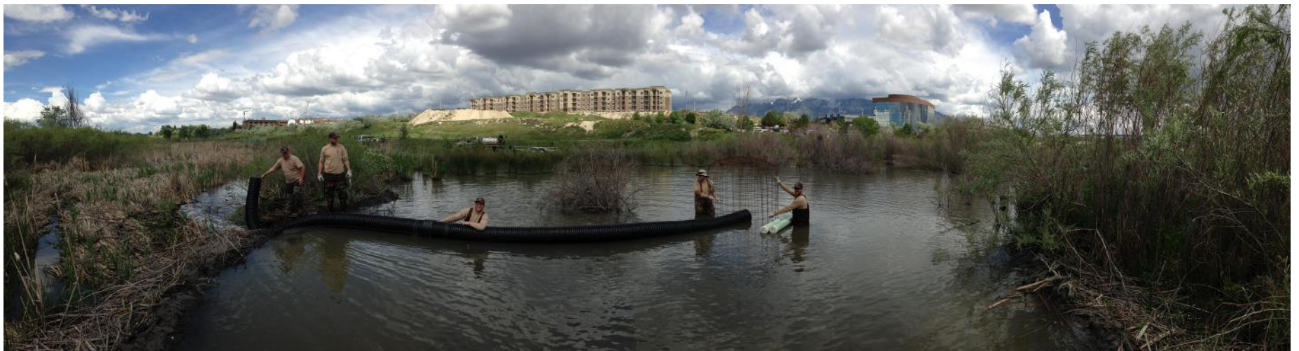
Utah Division of Wildlife Crew installing pond leveler on Jordan River Corridor property to manage beaver dam water levels. Photo courtesy Dave Lee
