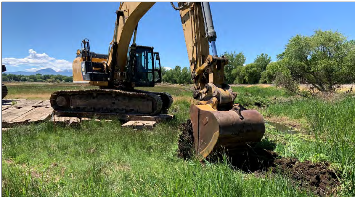
Ryan Proctor, U.S. Bureau of Reclamation, uses a backhoe stabilized on a "swamp mat" (a connected series of large timbers), to begin excavating the first channel in the delta restoration area in June 2020.
