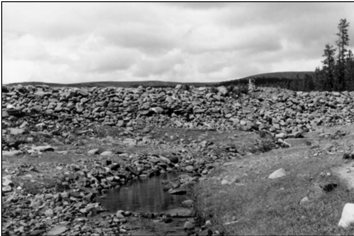
HAER UT-42-I. Island Lake Dam. Downstream face of dam; view to the north-northwest.
