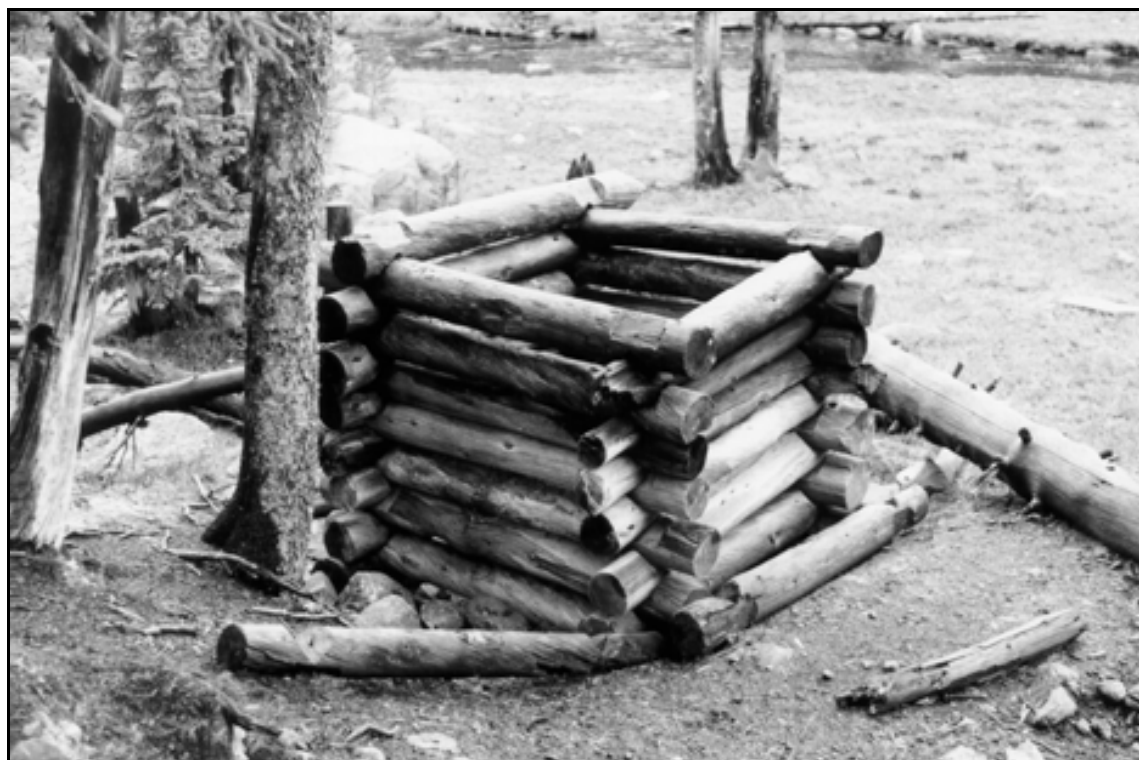
HAER UT-42-B. Brown Duck Lake Dam. Southeast corner of log privy foundation; view to the northwest.
