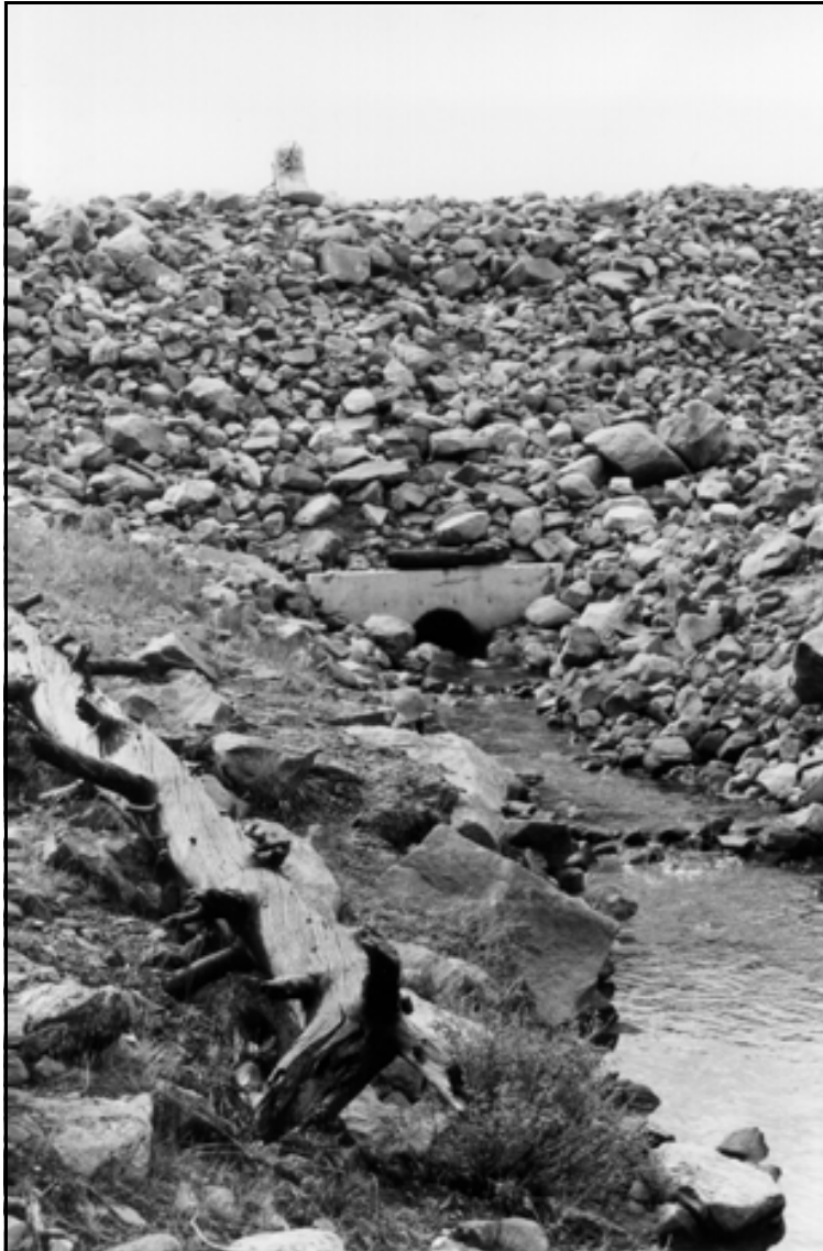
HAER UT-42-J. Kidney Lake Dam. Downstream face of outlet works; view to the west.
