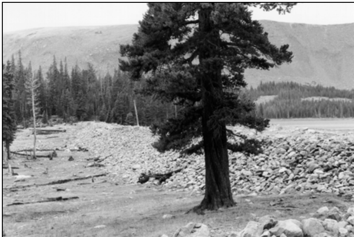
HAER UT-42-J. Kidney Lake Dam. Overview of dam; view to the southeast.
