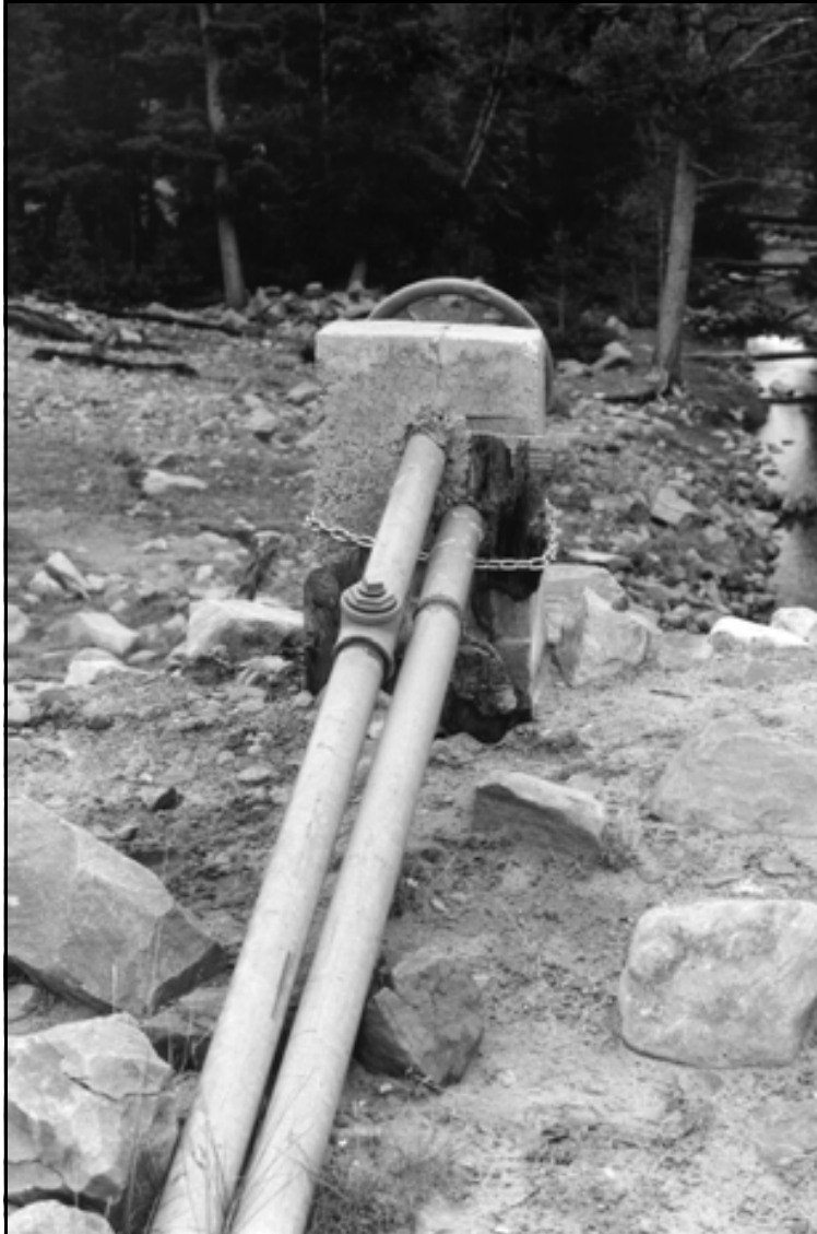
HAER UT-42-J. Kidney Lake Dam. Western face of canal gate handwheel pedestal; view to the east.
