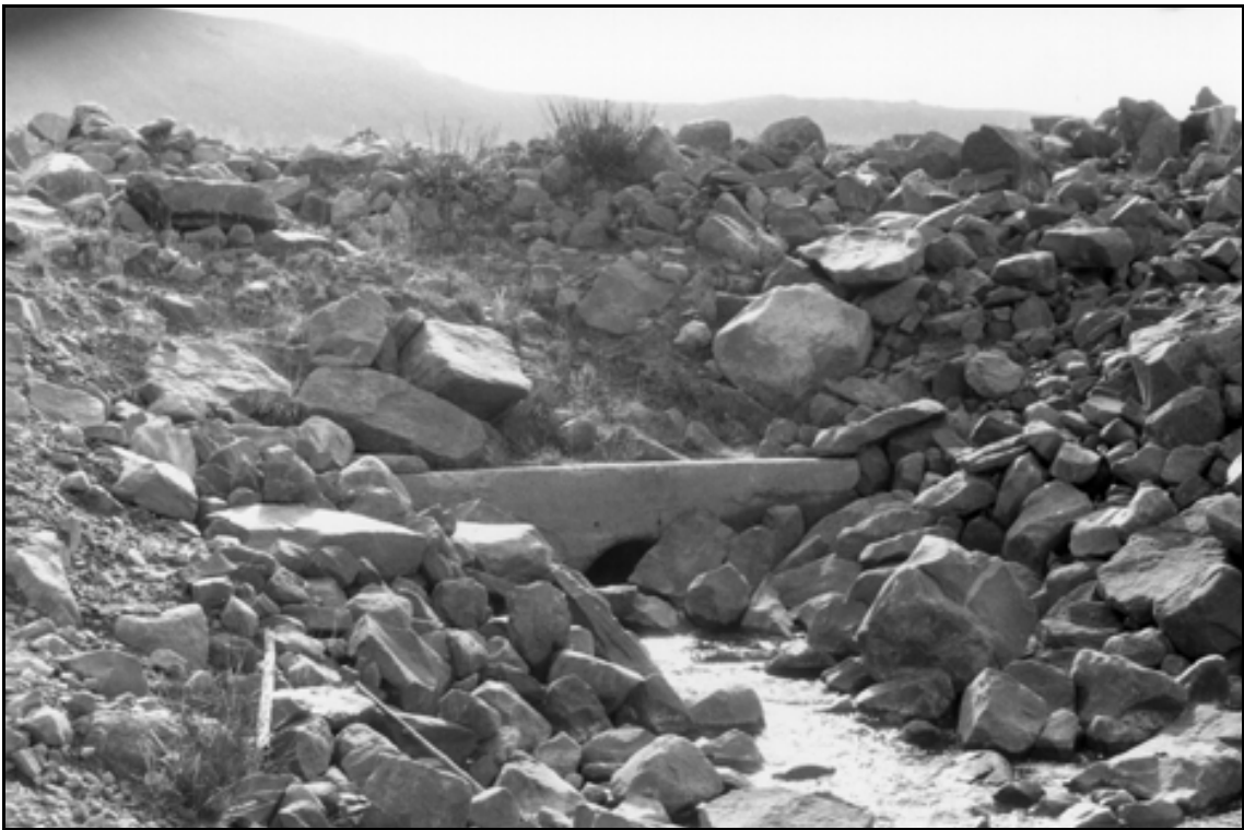
HAER UT-42-B. Brown Duck Lake Dam. Downstream face of outlet works; view to the west.
