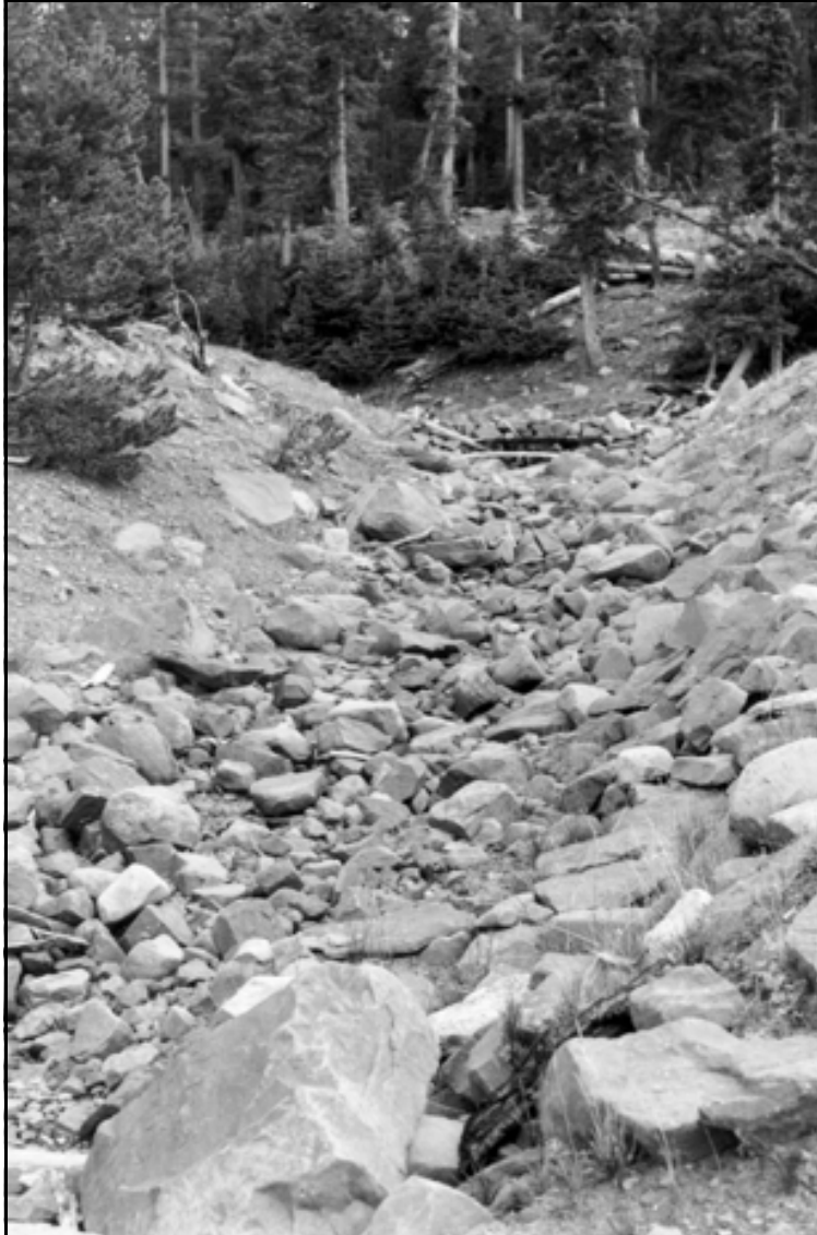
HAER UT-42-B. Brown Duck Lake Dam. Overflow spillway; view to the east-southeast.
