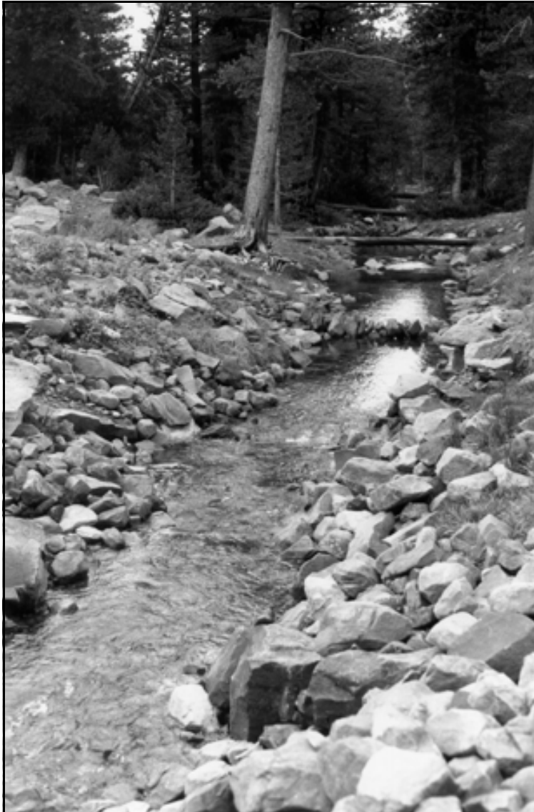
HAER UT-42-J. Kidney Lake Dam. Outlet spillway channel looking downstream; view to the east.
