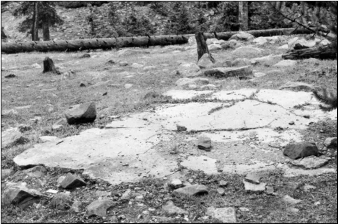
HAER UT-42-B. Brown Duck Lake Dam. Concrete pad; view to the north.
