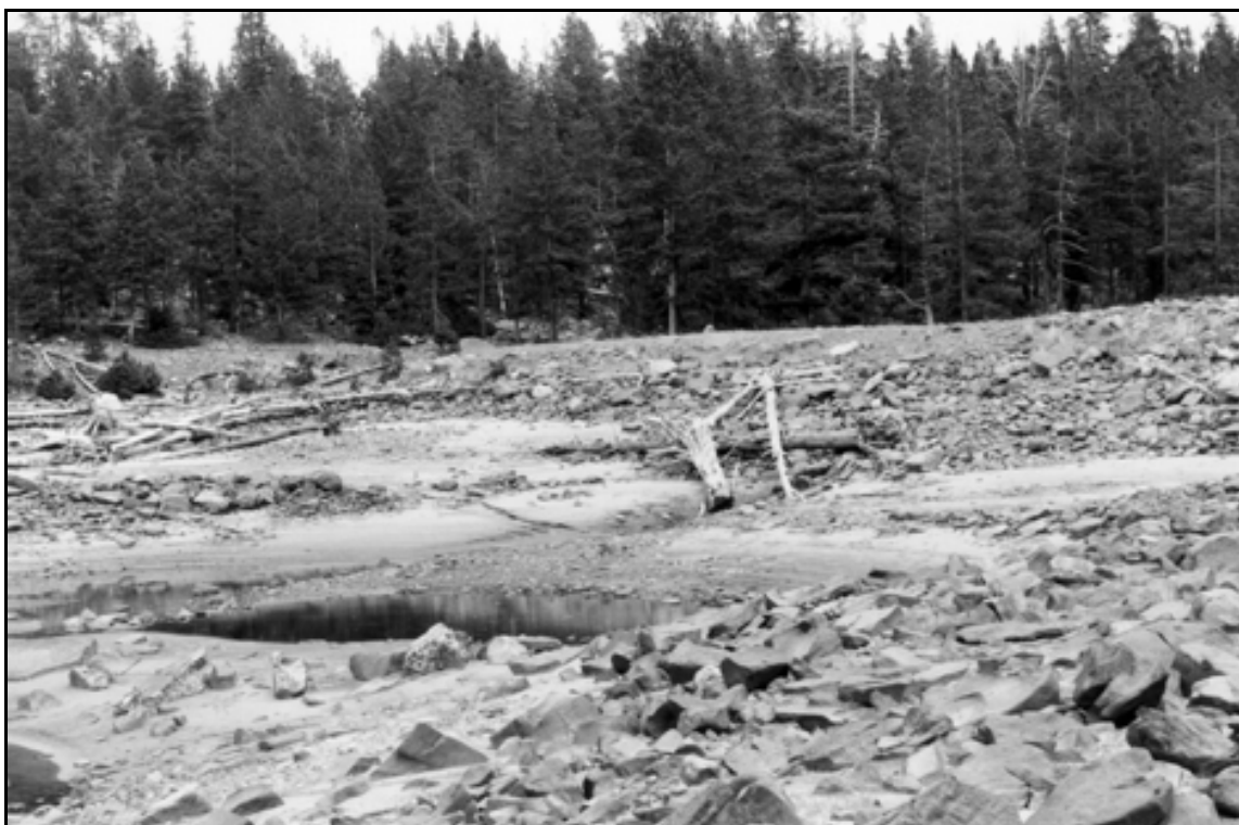
HAER UT-42-I. Island Lake Dam. Overview of dam; view to the south-southeast.
