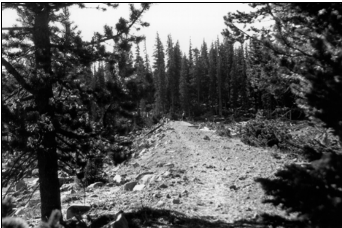
HAER UT-42-C. Clements Lake Dam. Overview of dam; view to the south.
