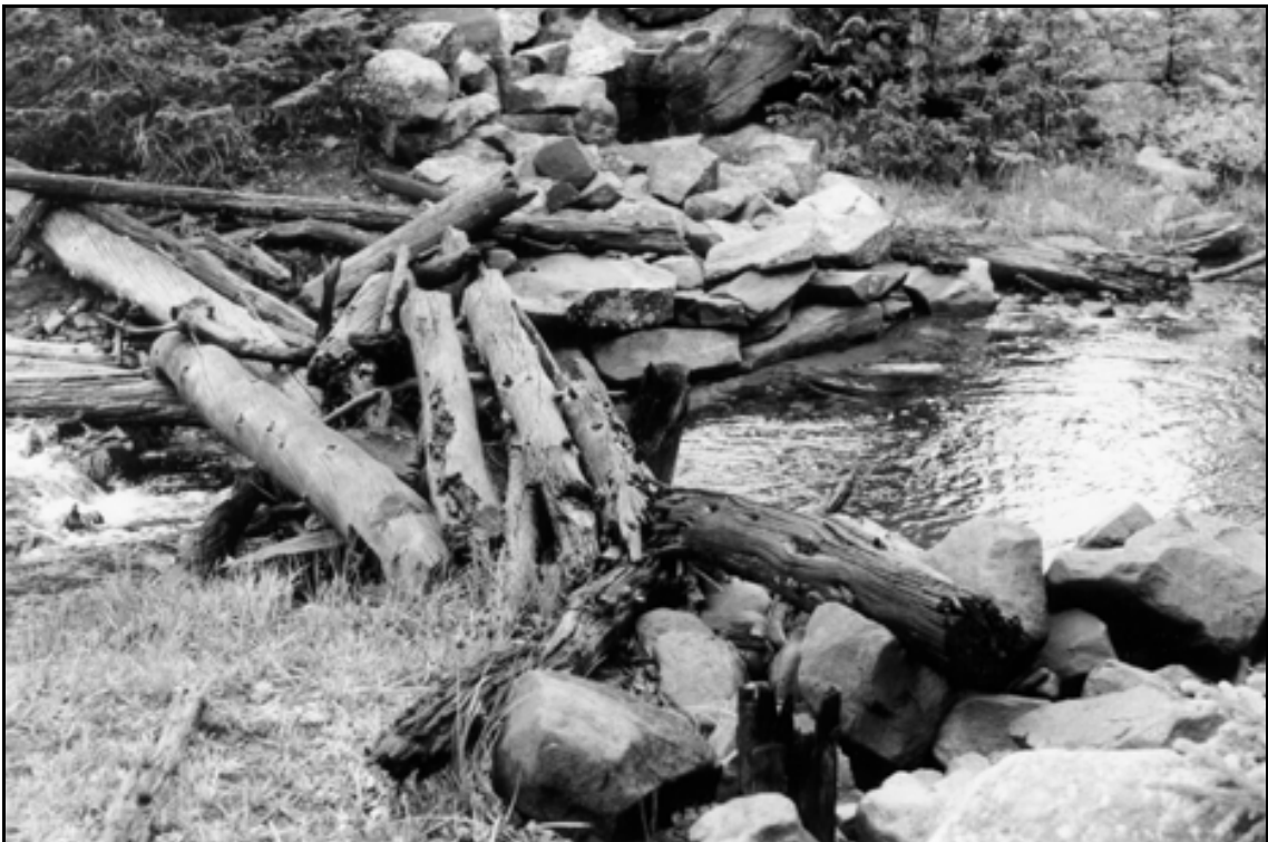
HAER UT-42-B. Brown Duck Lake Dam. Log check dam; view to the north.
