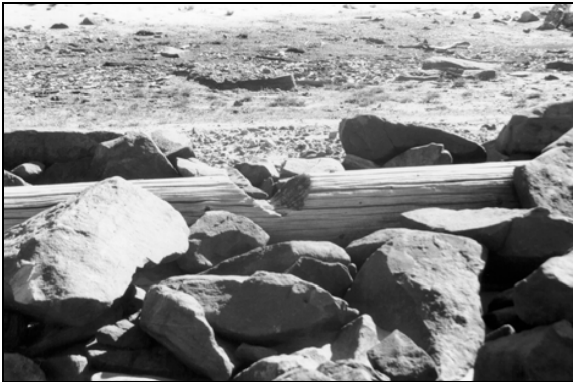
HAER UT-42-C. Clements Lake Dam. Notched log in shoring; view to the west-southwest.
