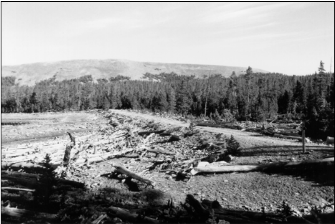
HAER UT-42-C. Clemens Lake Dam. Overview of dam; view to the north.
