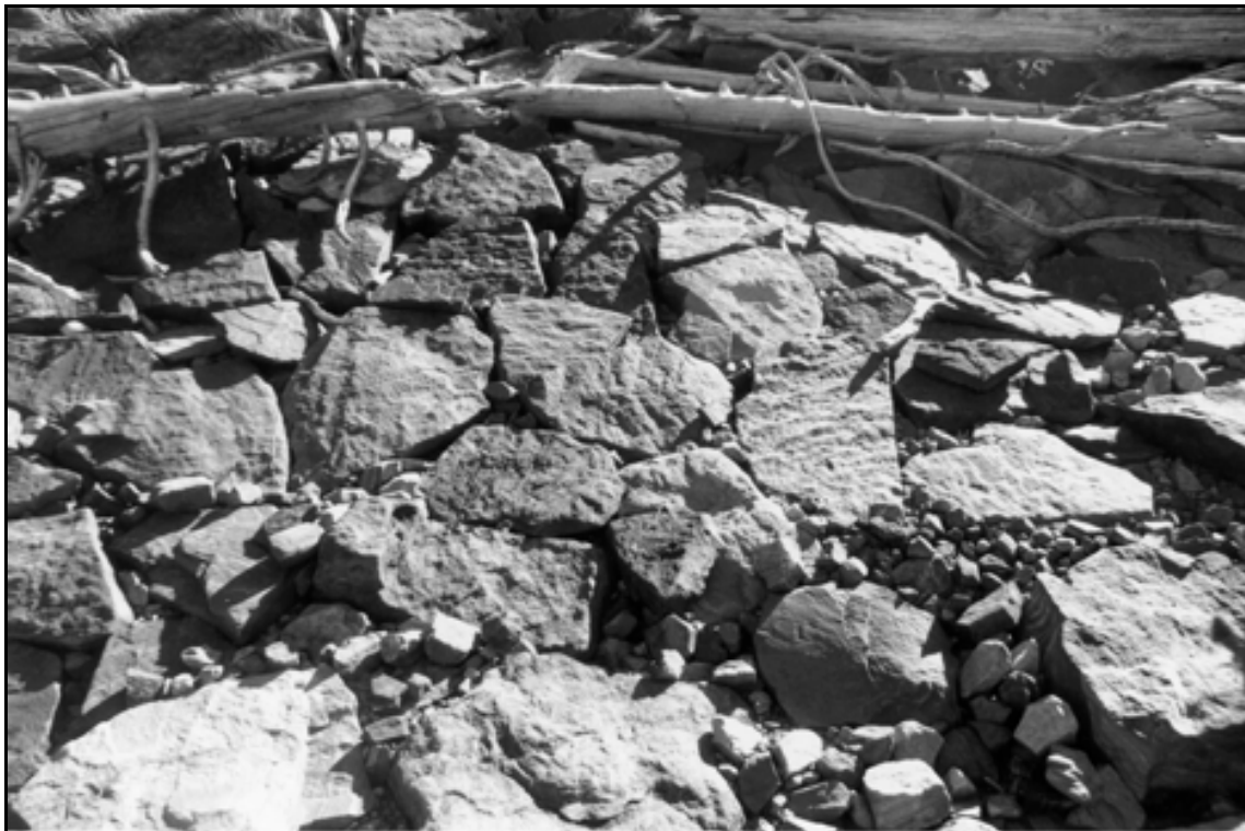
HAER UT-42-C. Clements Lake Dam. Tabular stone armorization; view to the west.
