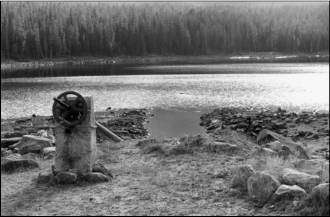
HAER UT-42-B. Brown Duck Lake Dam. East face of canal gate handwheel and pedestal; view to the west.
