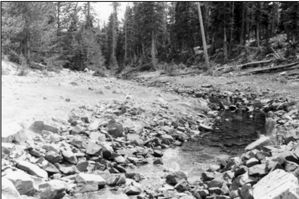
HAER UT-42-I. Island Lake Dam. Outlet spillway channel looking downstream; view to the south-southeast.
