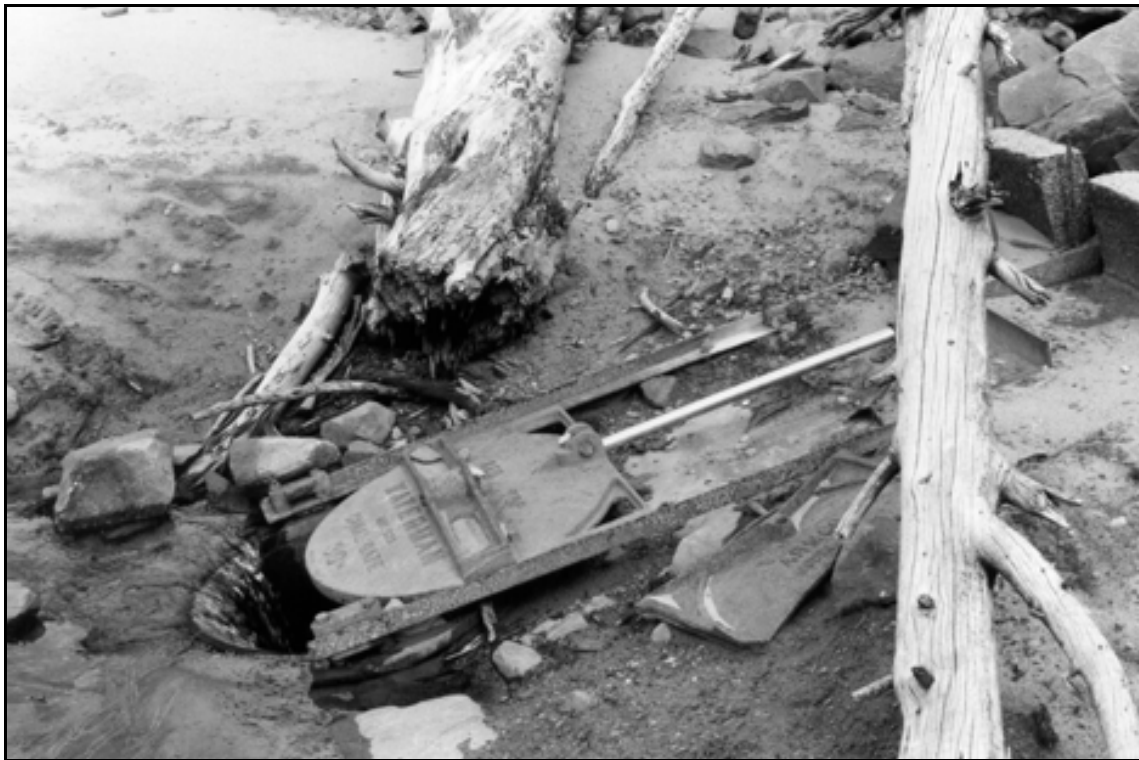
HAER UT-42-I. Island Lake Dam. Upstream face of outlet works; view to the east.
