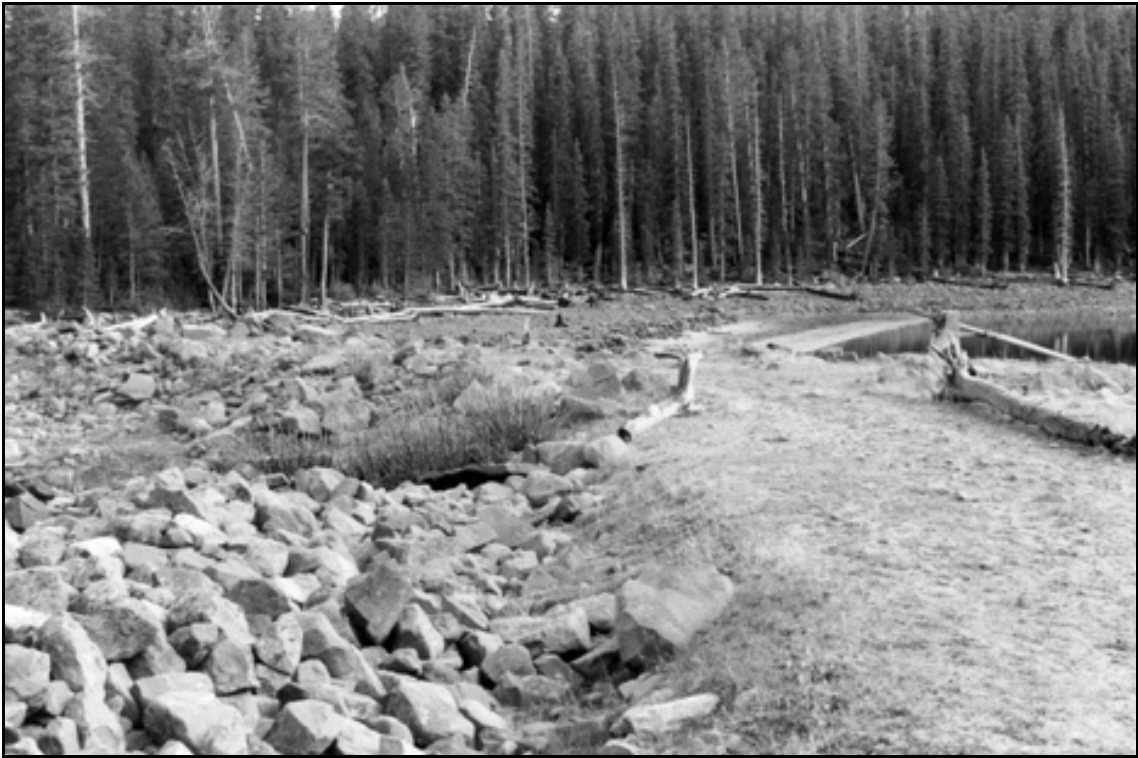
HAER UT-42-B. Brown Duck Lake Dam. Overview of dam; view to the north.
