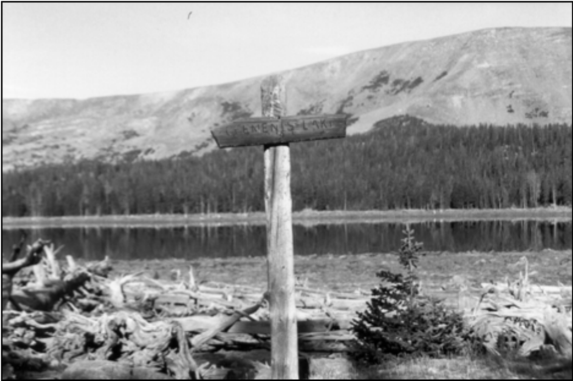
HAER UT-42-C. Clemens Lake Dam. Overview of Clemens Lake; view to the northwest.
