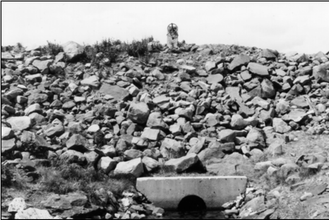
HAER UT-42-I. Island Lake Dam. Downstream face of outlet works; view to the west.
