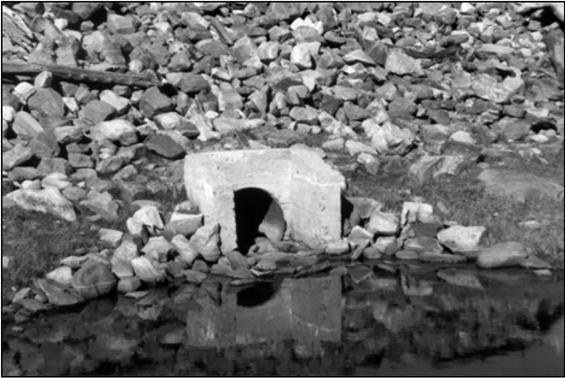
HAER UT-42-C. Clements Lake Dam. Downstream face of outlet works; view to the west-northwest.
