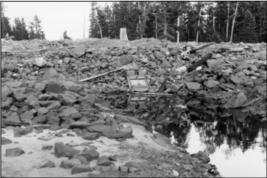
HAER UT-42-B. Brown Duck Lake Dam. Upstream face of outlet works; view to the east.
