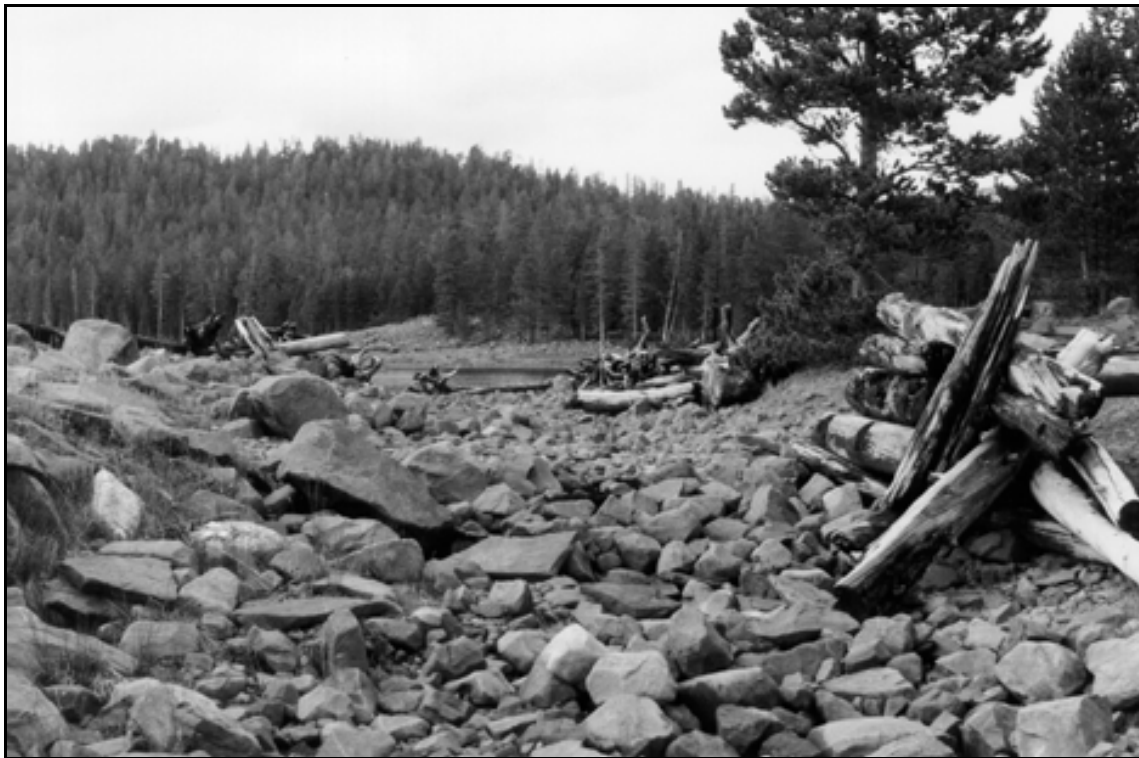
HAER UT-42-B. Brown Duck Lake Dam. Overflow spillway with notched logs; view to the northwest.
