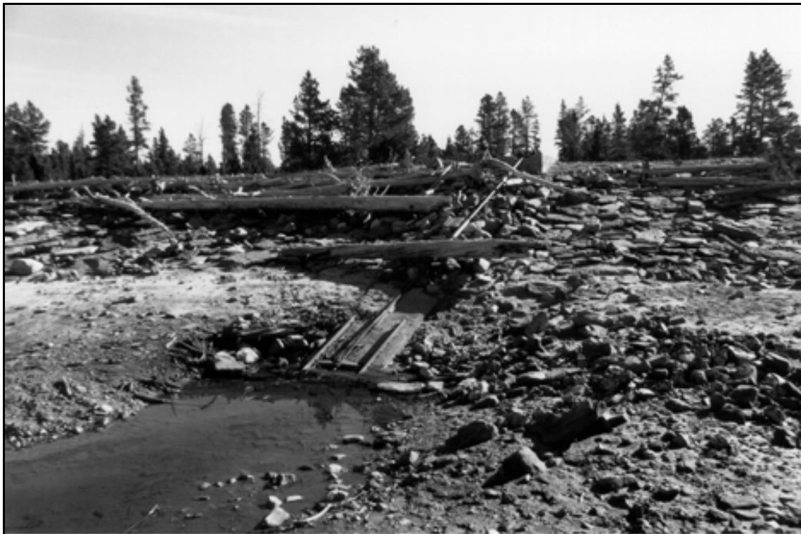
HAER UT-42-C. Clements Lake Dam. Upstream face of outlet works; view to the east-northeast.
