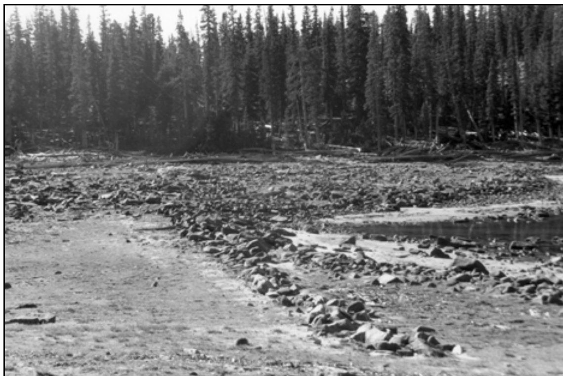
HAER UT-42-C. Clements Lake Dam. Overview of shoring; view to the south.
