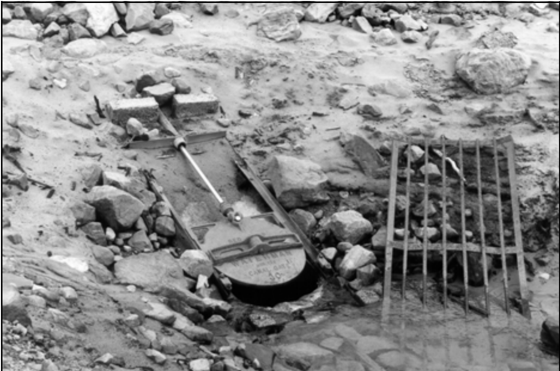
HAER UT-42-J. Kidney Lake Dam. Upstream face of outlet works; view to the east.
