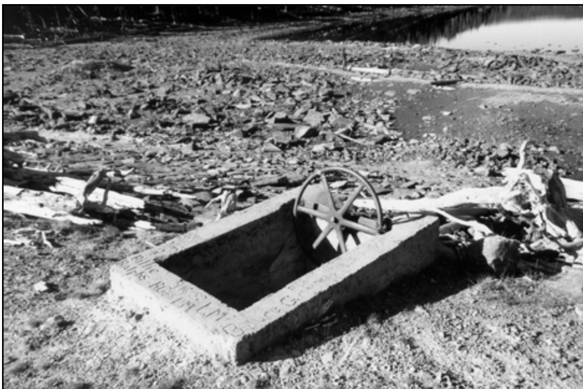
HAER UT-42-C. Clements Lake Dam. Northeast corner of canal gate handwheel box; view to the southwest.
