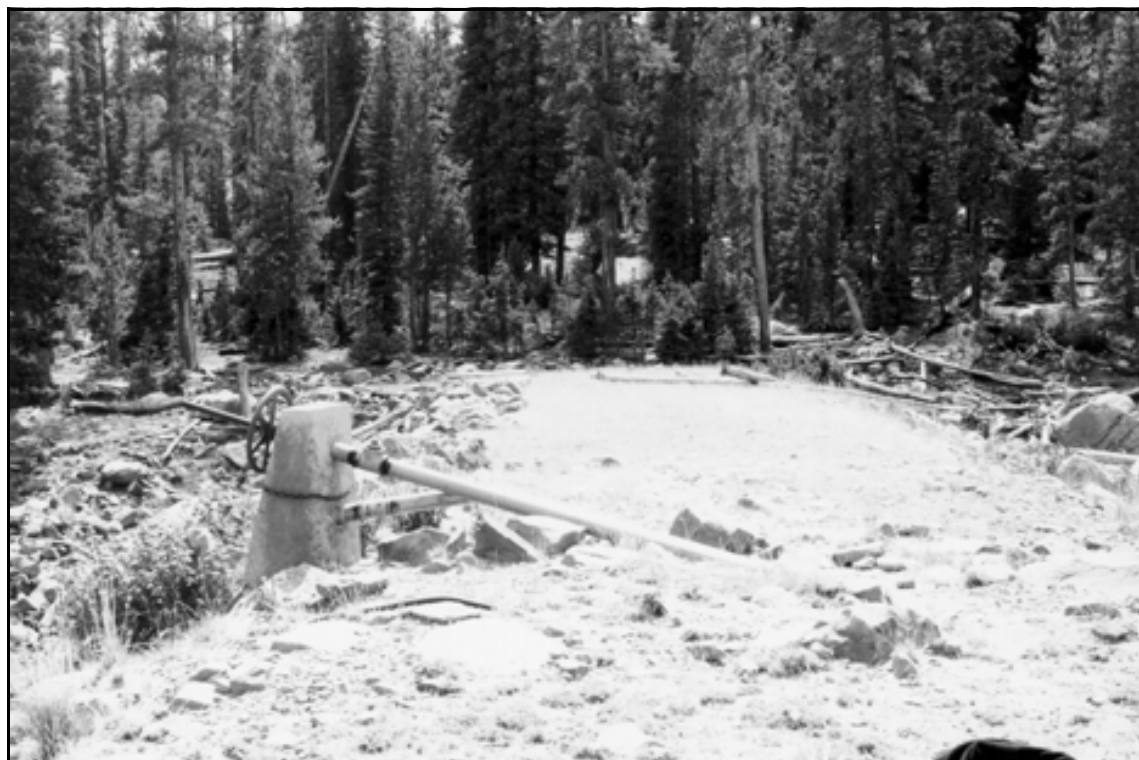
HAER UT-42-I. Island Lake Dam. North face of canal gate handwheel pedestal; view to the south.
