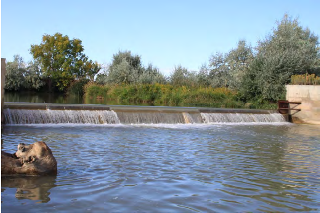
Myton Townsite Diversion
