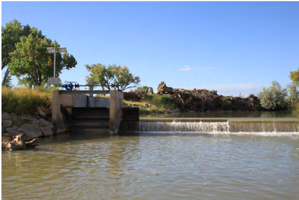
Myton Townsite Diversion
