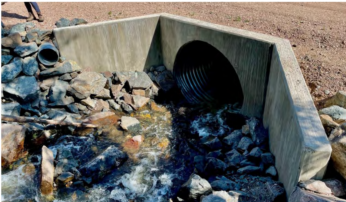
Properly sized and placed culvert
