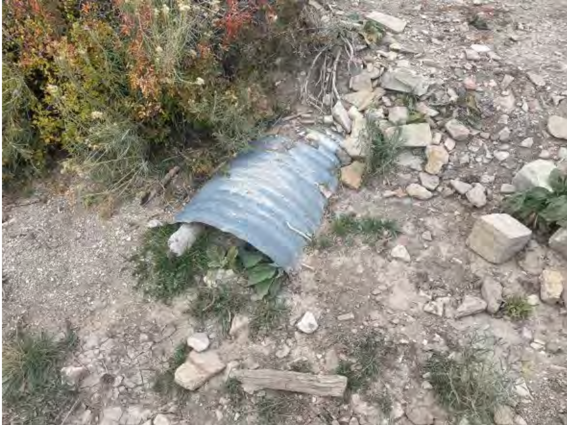
Photo 5. Example of a clogged culvert
