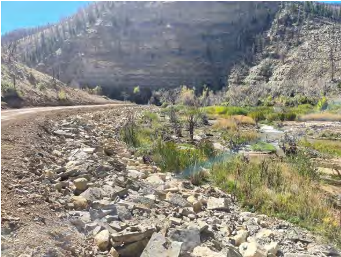
Photo 17. Riprap currently located along the Strawberry River Road.
