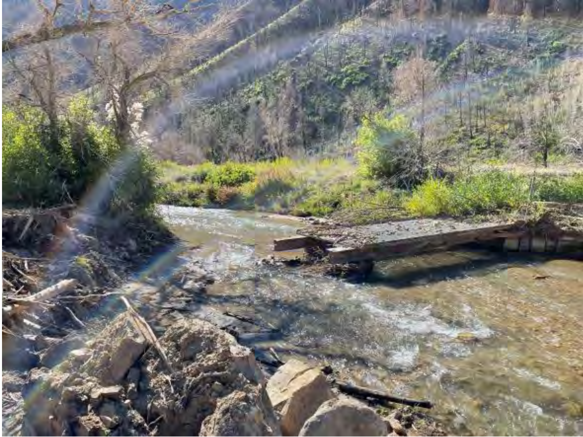
Photo 15. Bridge blowout at mile 8.1 (2021)
