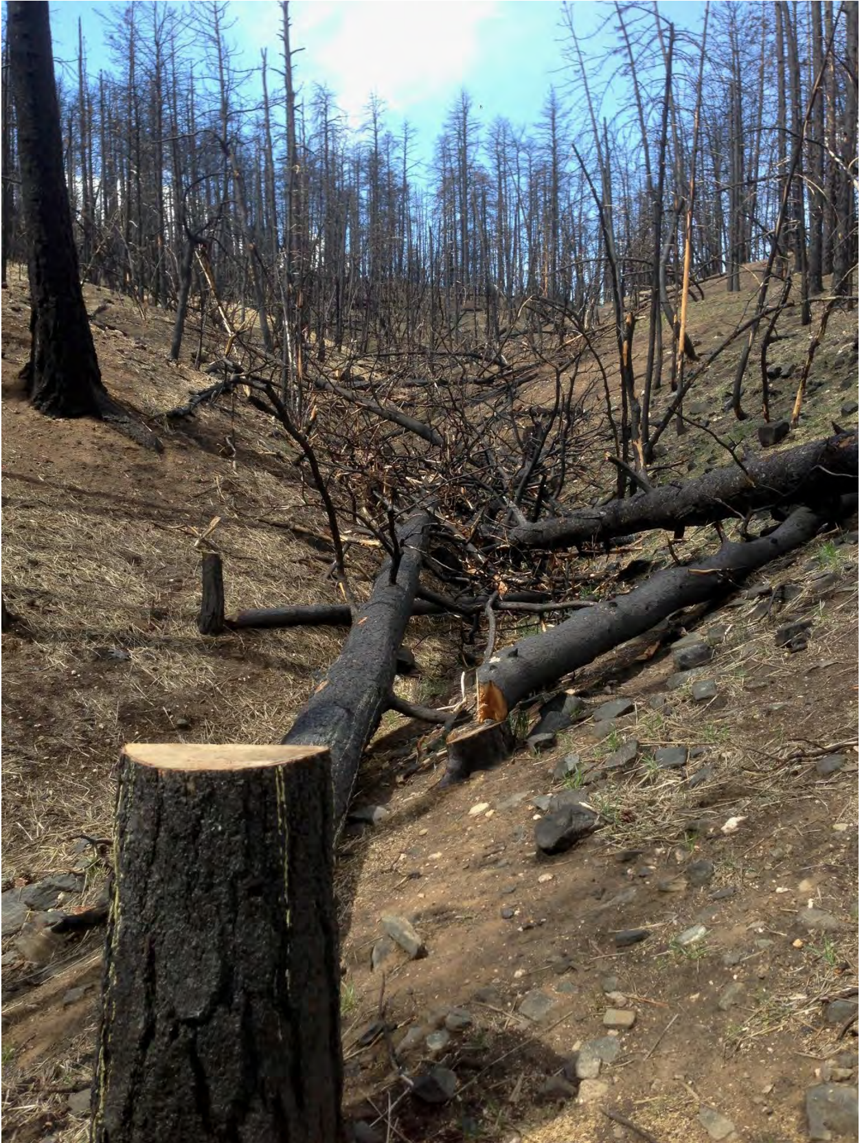
Felled trees placed for gully stabilization
