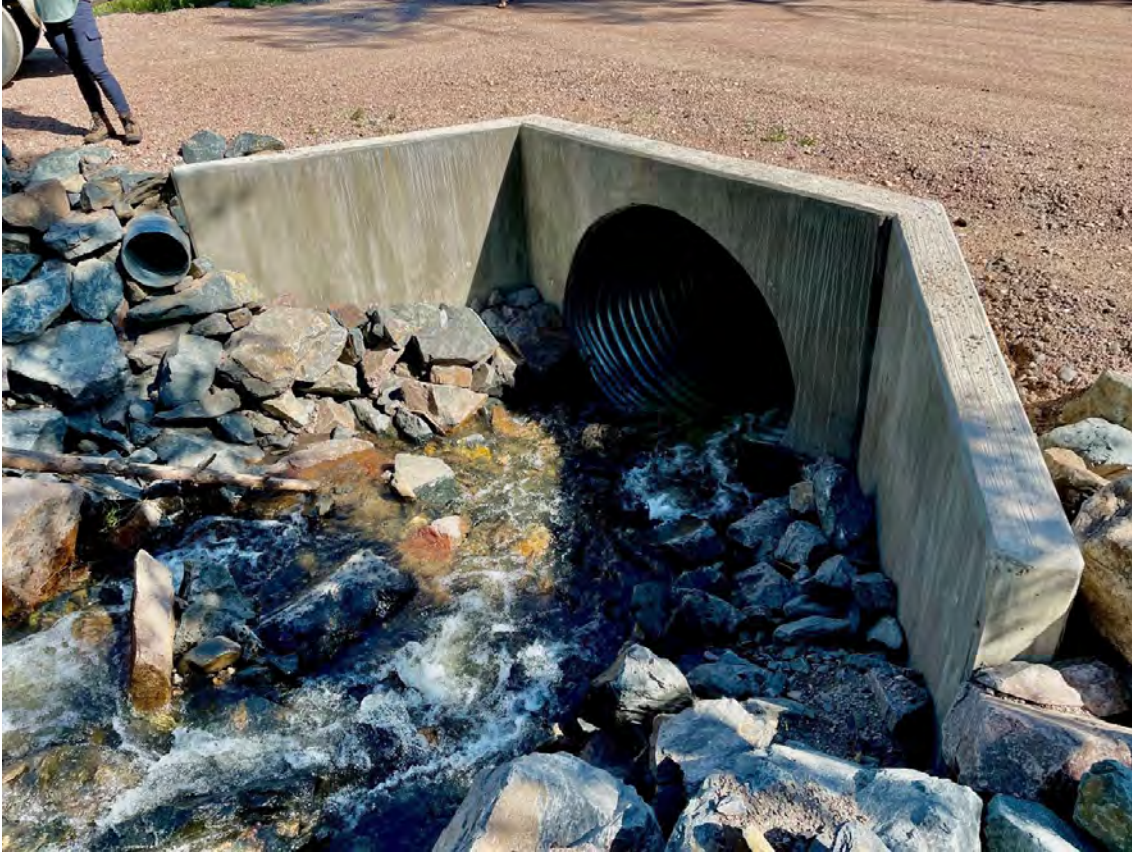
Photo 6. Properly functioning culvert
