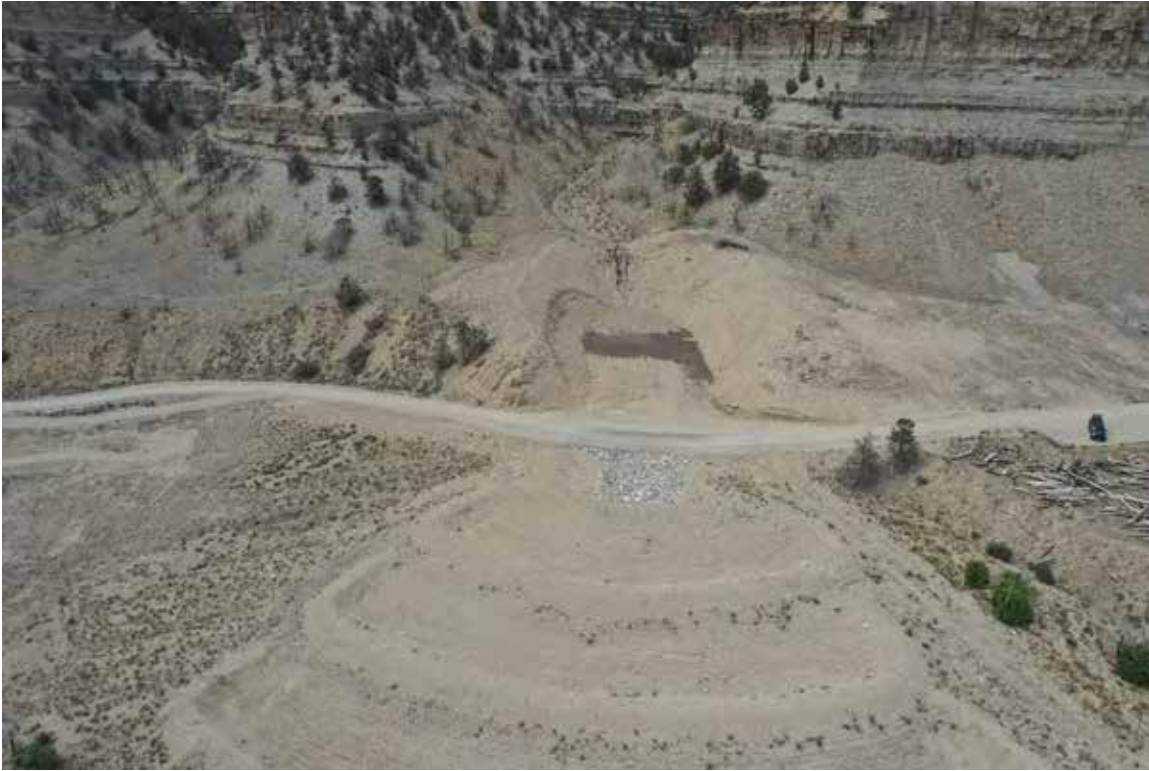
Figure 2.7. Alluvial fan that was excavated as part of EWP actions. The intermittent basin that created this fan has a drainage area of 1.8 square kilometers.
