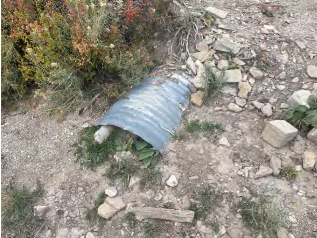
Figure 2.9. Example of a clogged culvert
