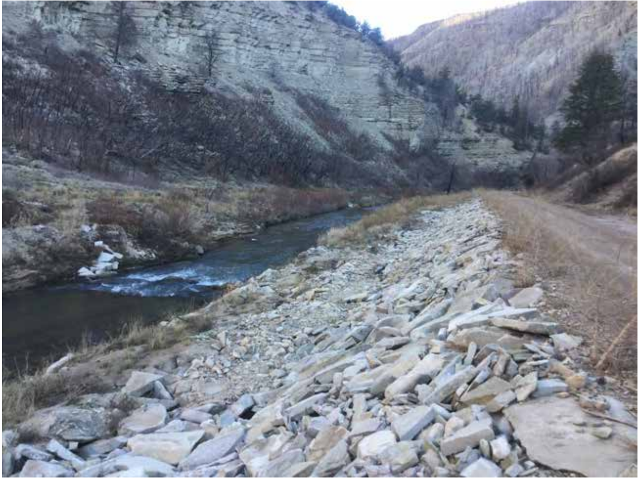
Figure 3.48. River Km 22.25-23.5. The channel is confined by the road and valley margin with rip-rap in several locations. Because geomorphic changes are limited here, only structure additions are recommended to increase habitat complexity.
