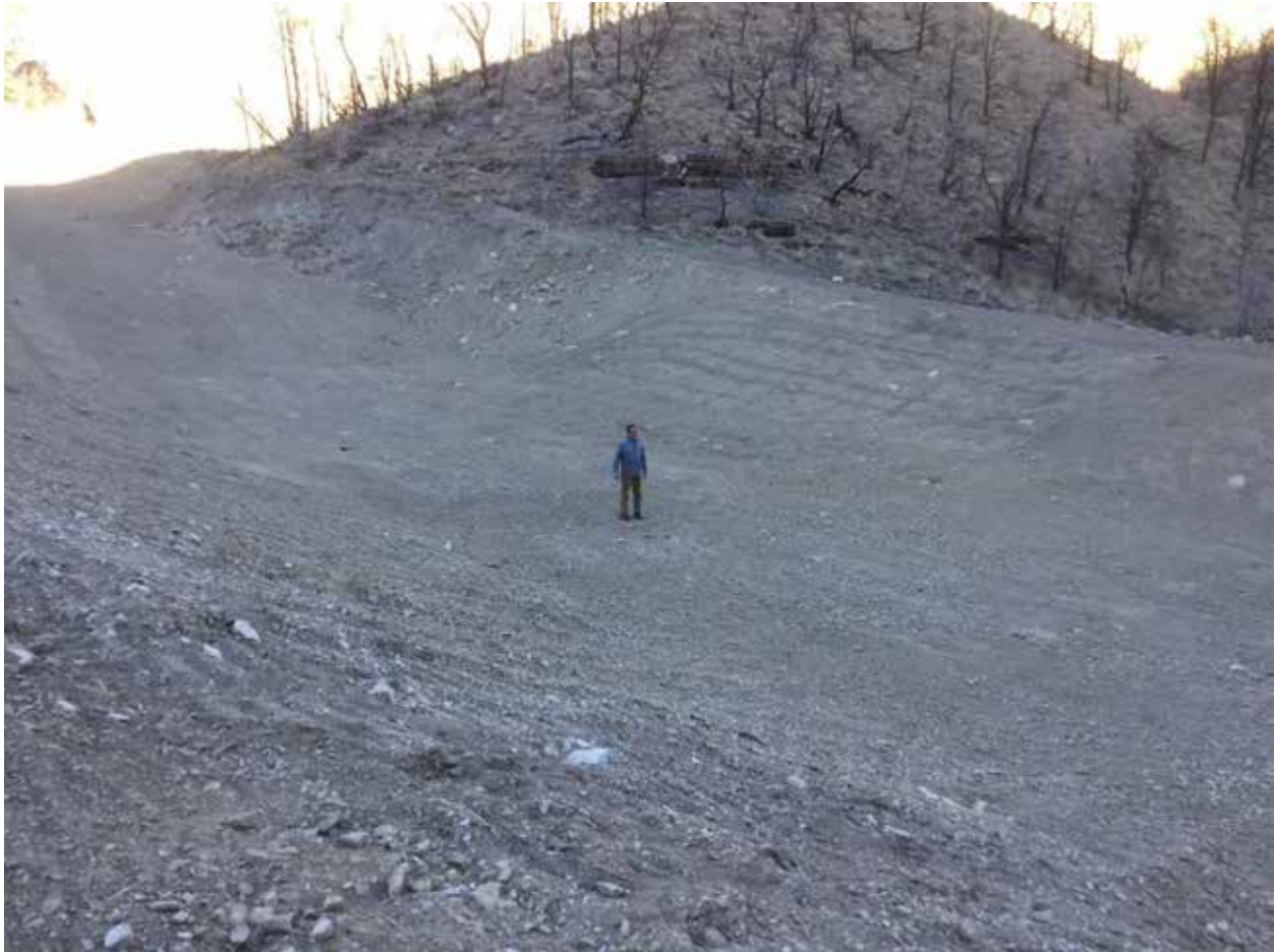
Figure 10.1. Excavated alluvial fan along the Strawberry River. The basins excavated from alluvial fans range in size. The one pictured here is approximately 40 yards wide and 50+ yards long and excavated to depth of roughly 5 yards.
