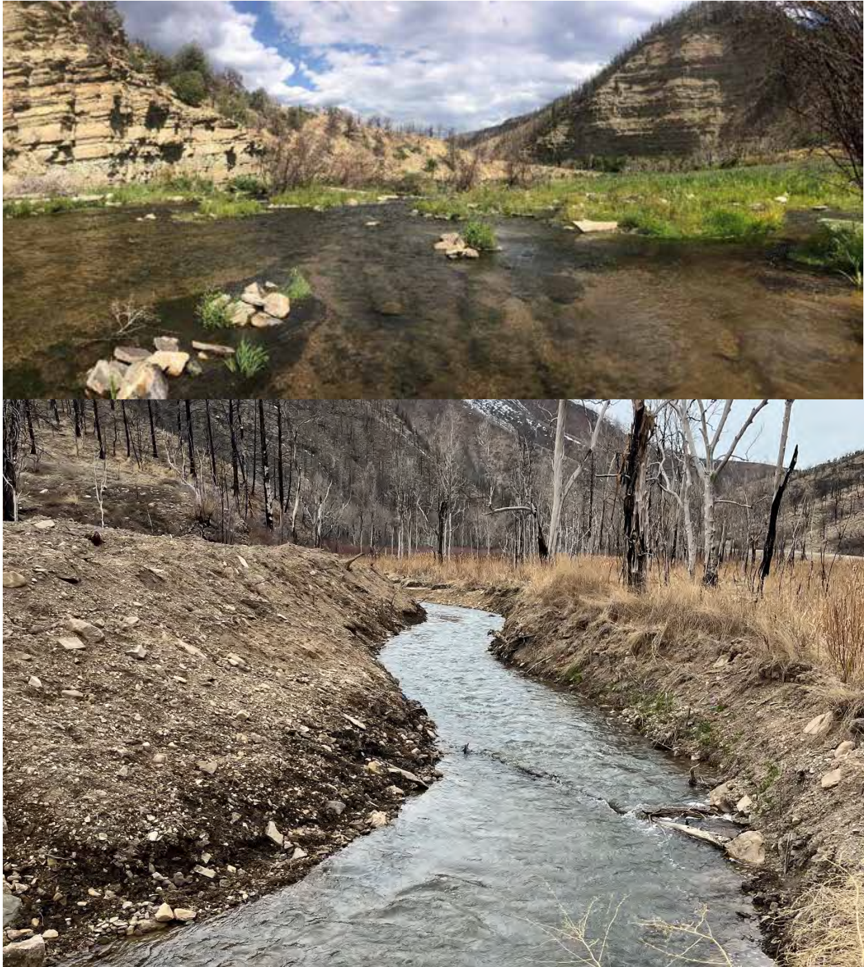
Figure 3.44. River Km 19.25-22.25. A debris flow out of Timber Draw created an alluvial fan that dammed the mainstem Strawberry resulting a complex multi-threaded channel (top photo). The channel was simplified to a single-threaded highly entrenched channel (bottom photo) as part of the EWP work created to drain the large pond above the alluvial fan. Structures will need to be added to the channel to increase complexity.
