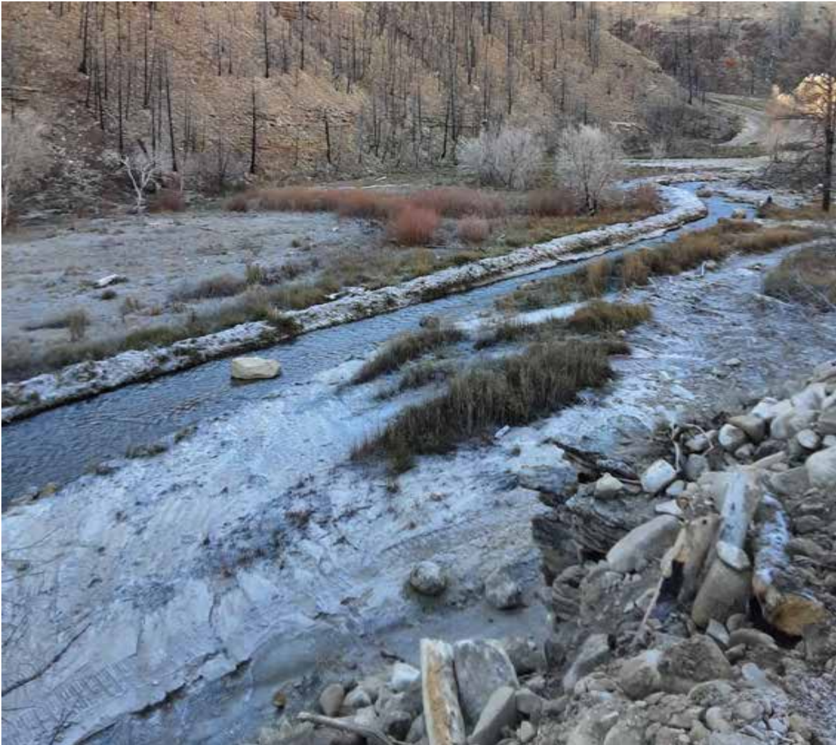
Figure 3.41. River Km 18.5-18.75. EWP modified narrow straighten channel below Sulphur Draw. Note levee on the river right side of the channel (water right to left). Levee removal, new channels in the floodplain, and structures will allow frequent inundation of the floodplain that will support riparian plantings.
