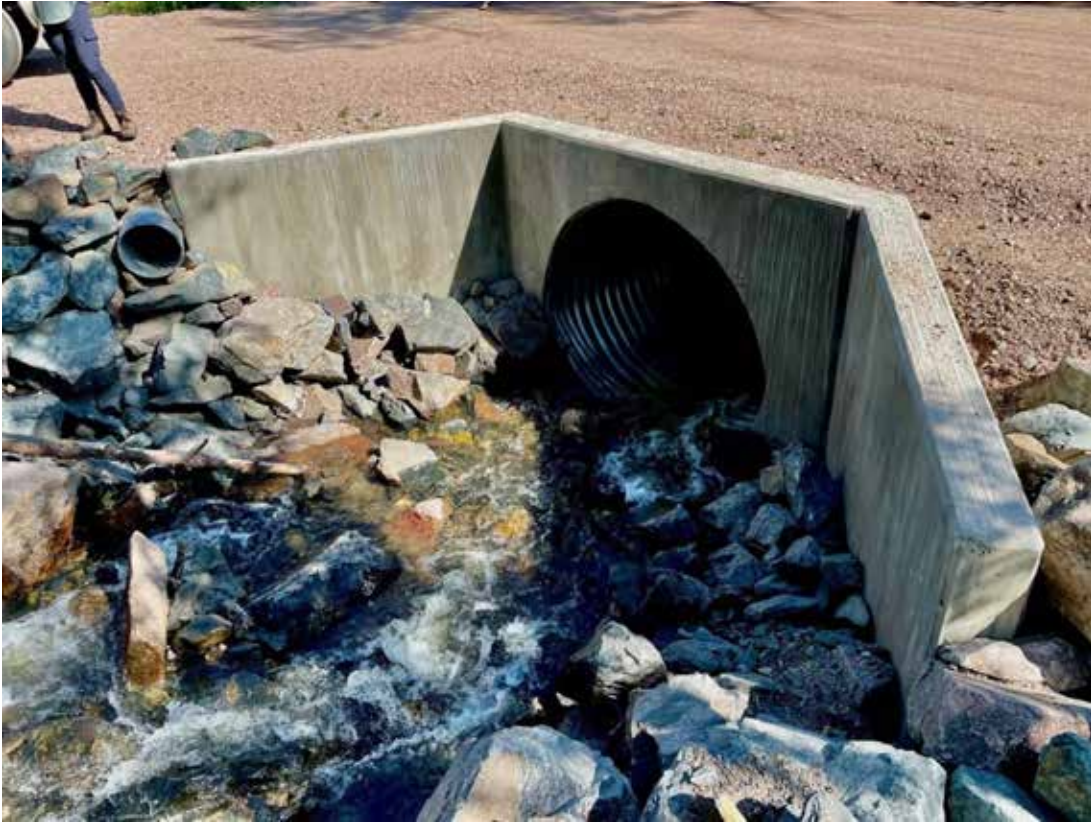
Figure 2.10. Properly functioning culvert
