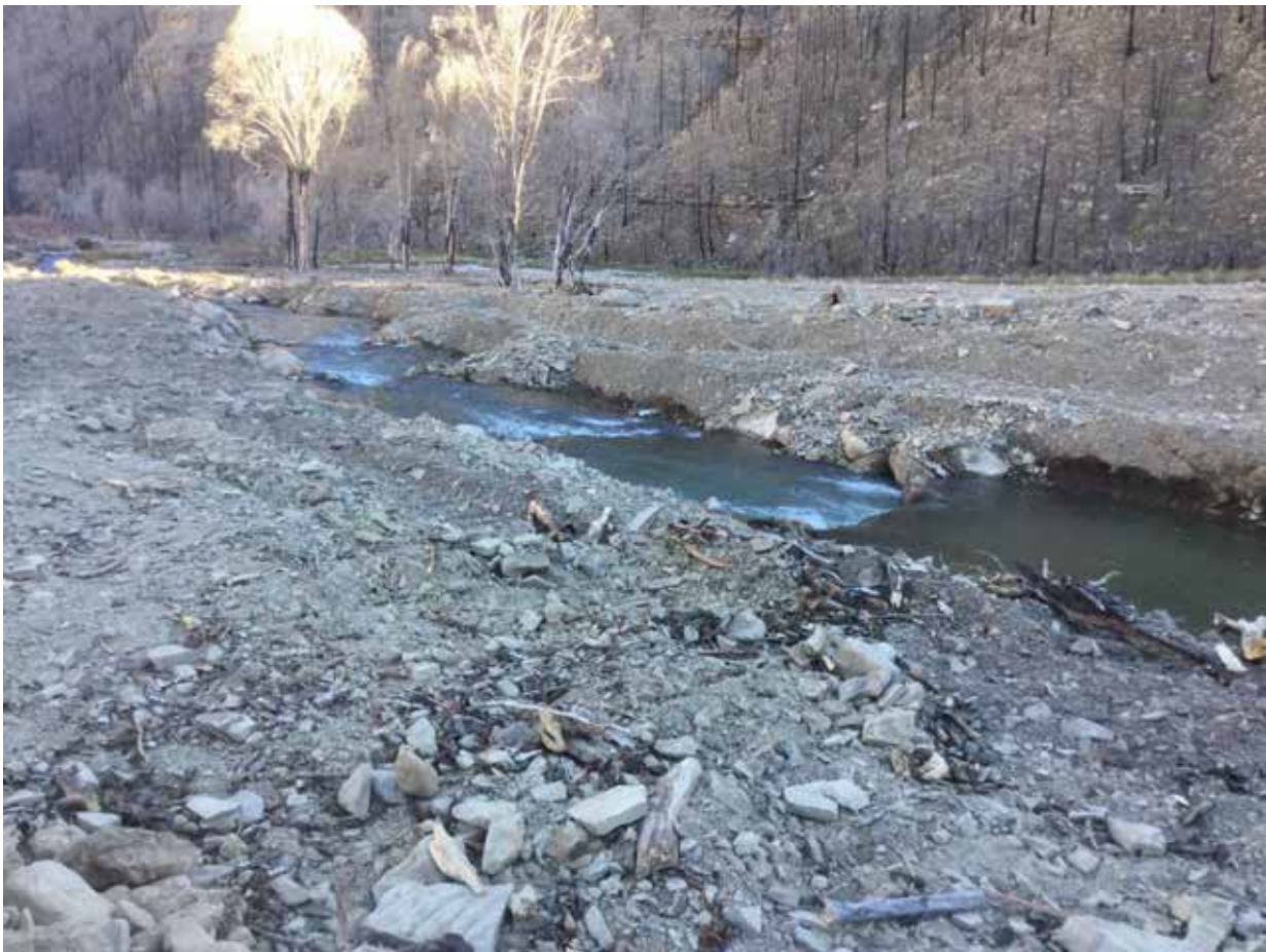
Figure 3.18. Recently constructed single-thread high-entrenchment (due to material deposited on the bank during channel straightening) channel with instream structures.
