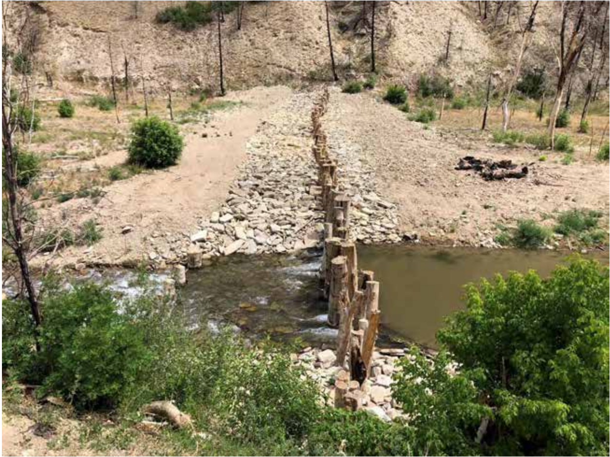
Figure 3.24. Debris catcher near River km 28.5. This structure extends laterally across the valley bottom and can capture wood mobilized from upstream reaches, protecting downstream infrastructure.
