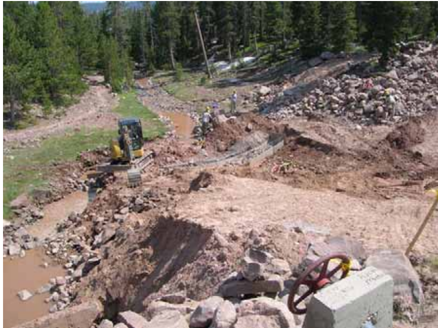
Figure 23: Installation of the downstream gabion basket cut-off wall.
