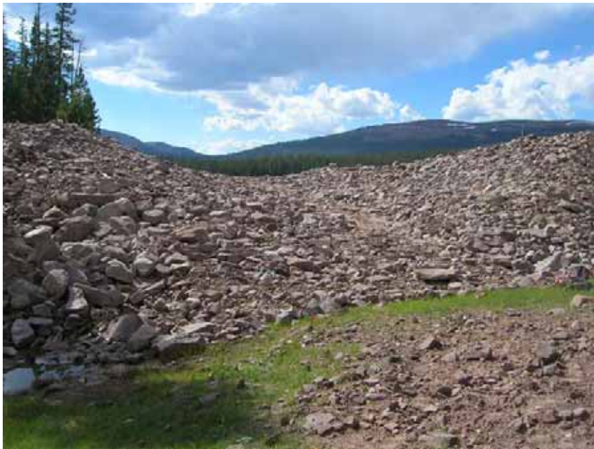
Figure 30: Looking upstream to the completed breach at Island Lake.
