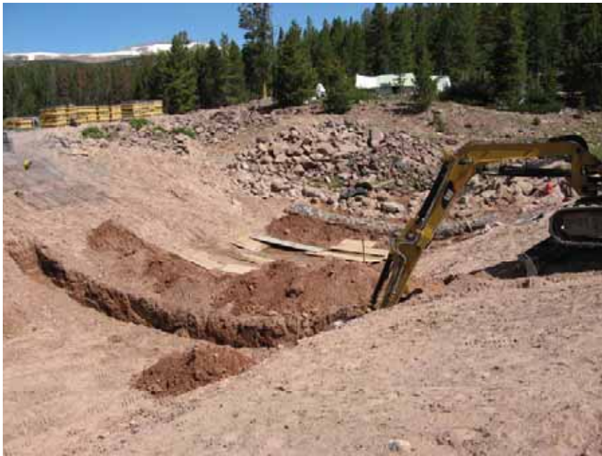
Figure 9: Installation of the middle cut-off wall.
