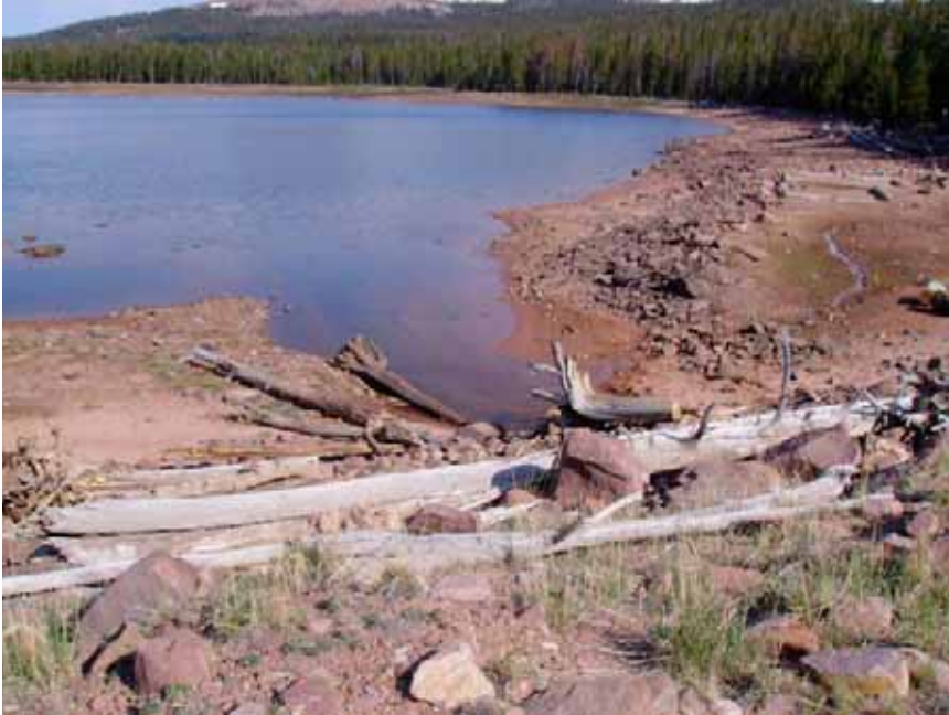
Figure 19: Dam inlet and upstream face of dam at start of project. UCC crew used cross-cut saws to cut and remove dead logs from dam.
