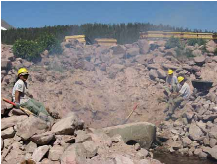
Figure 10: UCC crew used heat from burning logs removed from the shoreline to crack the concrete and then break up the materials with hand tools. The crew had only marginal success with this method.
