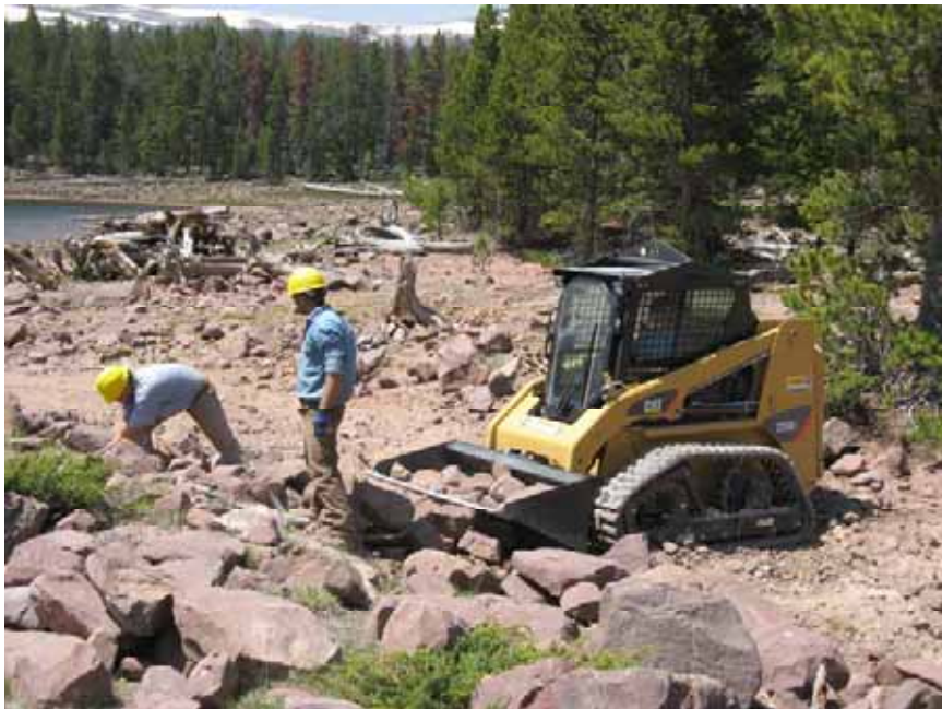
Figure 4: Crew working on gathering rock for gabions.
