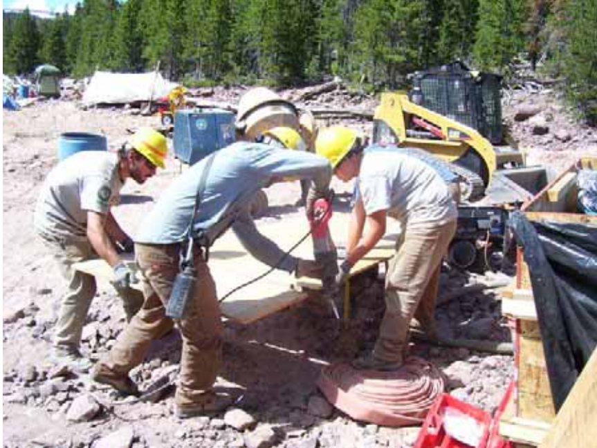
Figure 27: UCC crews cutting up forms for the outlet grouting operation.
