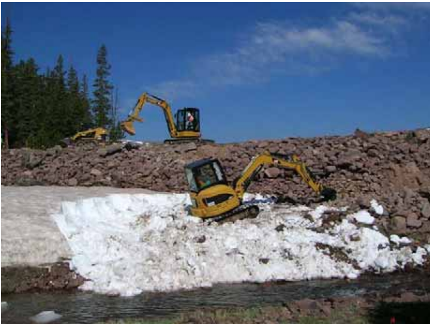
Figure 20: Snow and riprap removal during beginning stages of construction by BOR crew.
