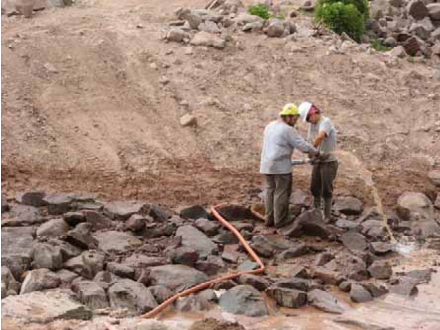
Figure 12: UCC crew washing fines down the bottom of channel.
