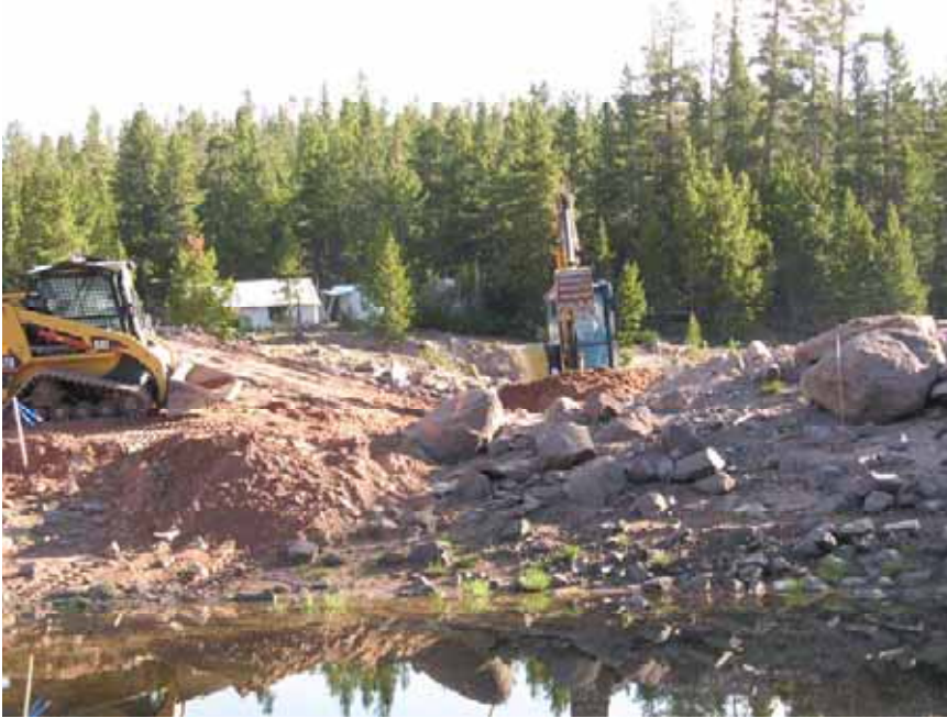
Figure 6: Crew continued cutting through dam using mini-excavator and skid steer.
