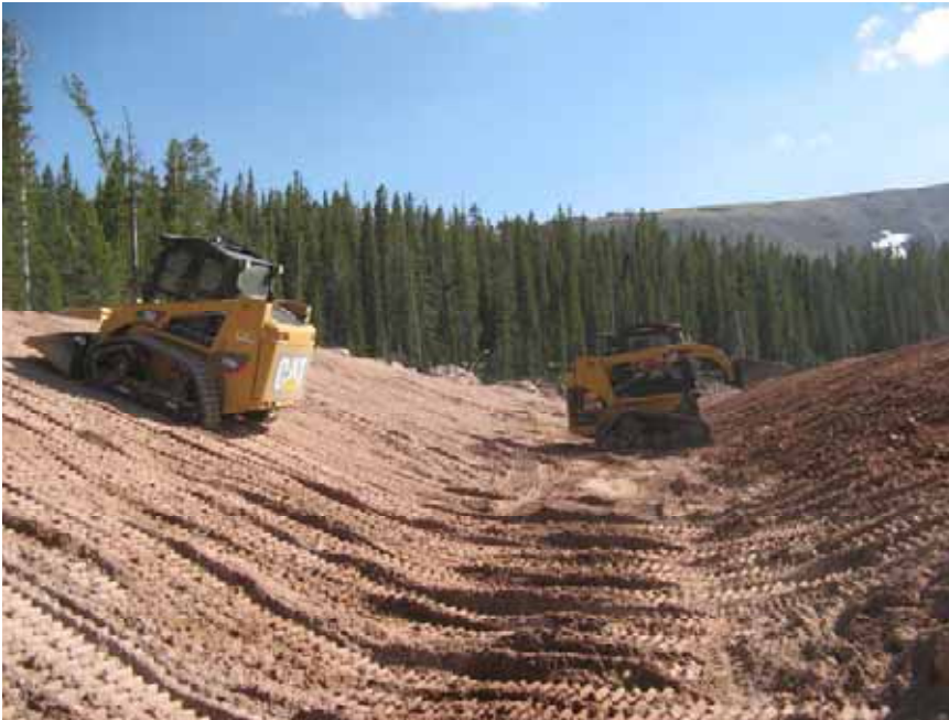
Figure 7: View of breach completed prior to placing cut-off walls and riprap.
