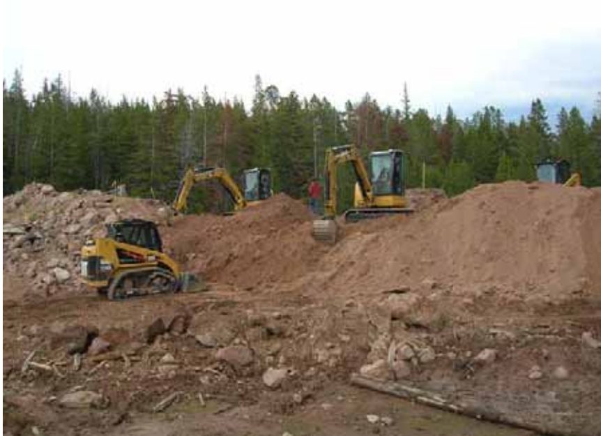
Figure 21: Initial excavation through the dam.
