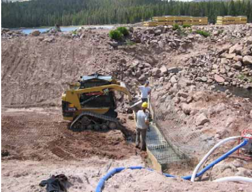
Figure 8: UCC crew helping with installation of gabion baskets at downstream cut-off wall.
