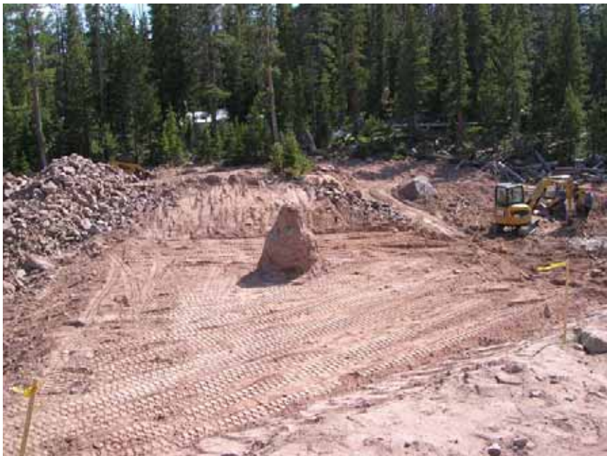
Figure 22: Excavating through the dam embankment with center stake still in place.
