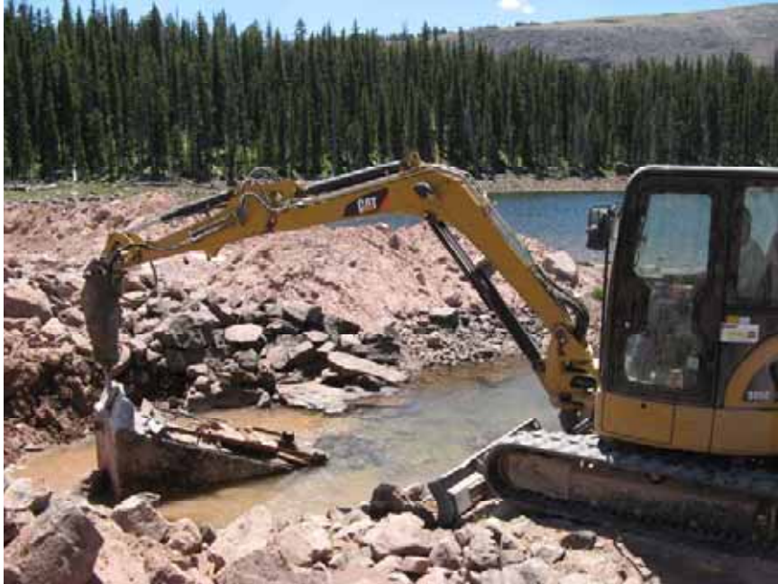
Figure 13: Demolition of inlet structure using stinger attached to trackhoe.
