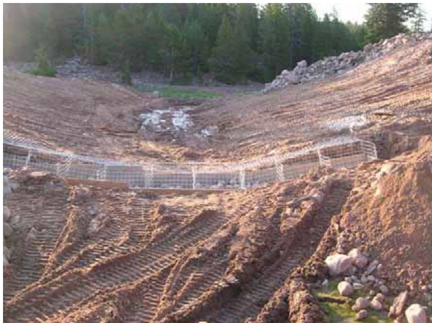
Figure 24: Installation of the upstream cut-off wall.
