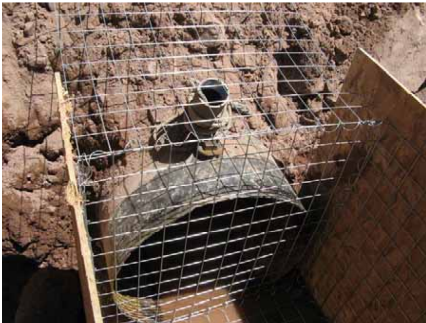
Figure 14: Gabion basket installed at each end of outlet pipe to be filled with rock and grout.
