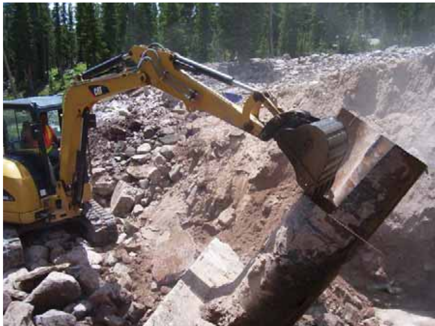
Figure 26: Removal of outlet structure and pipe prior to grouting.
