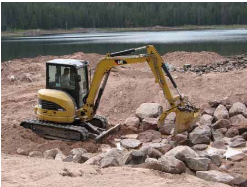
Figure 11: Crew placing riprap in the channel.
