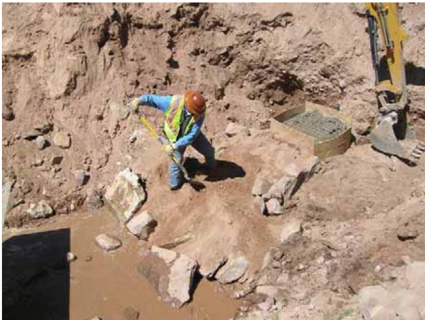
Figure 28: Grouted pipe and sand filter installed on downstream side of existing outlet.
