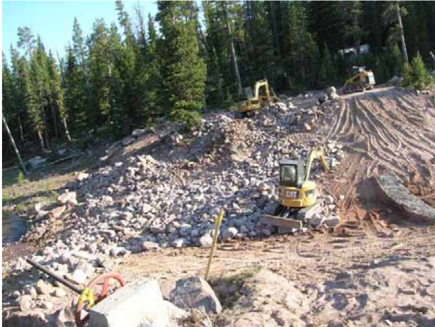
Figure 25: Riprap placement using mini-excavators and front loaders.
