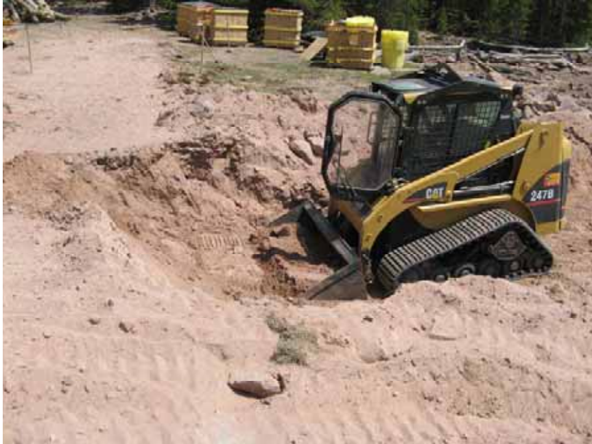
Figure 5: DCWCD crew using skid steer to begin cutting breach through the Dam after riprap was removed.
