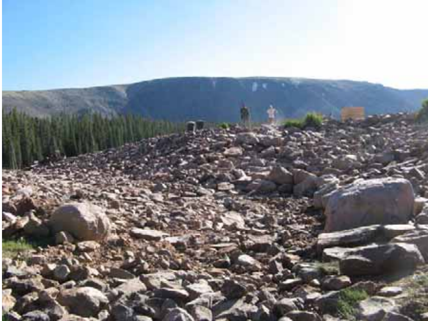
Figure 16: Looking upstream to the completed breach channel at Brown Duck Lake.
