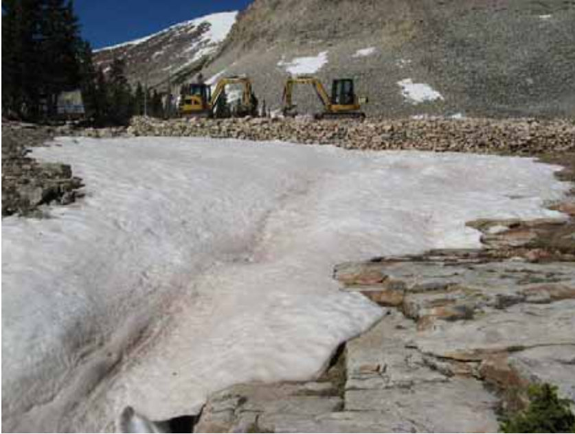
Figure 28: Crews working to remove the snow drift below dam at Drift Lake.
