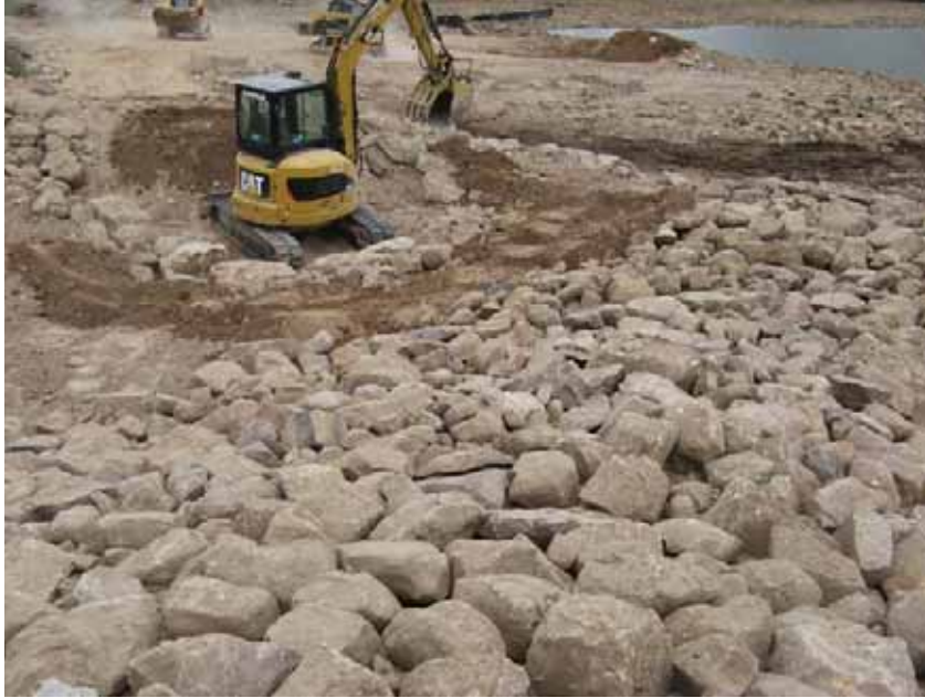
Figure 18: Crew placing riprap in the channel using mini-excavator.
