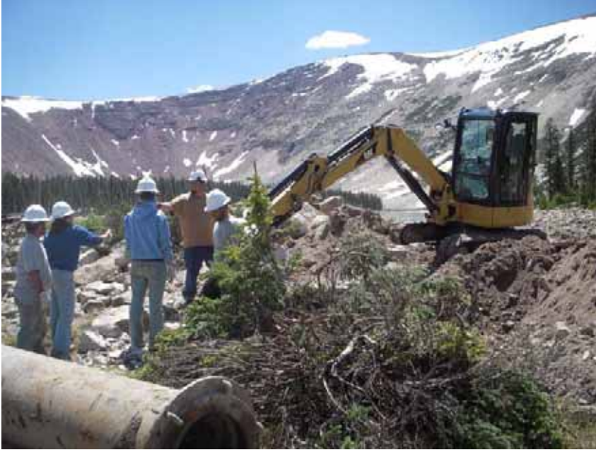
Figure 24: Crew removing outlet pipe.
