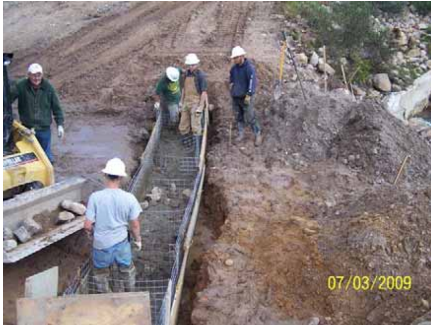
Figure 10: Installation of the middle cutoff wall at Five Point.
