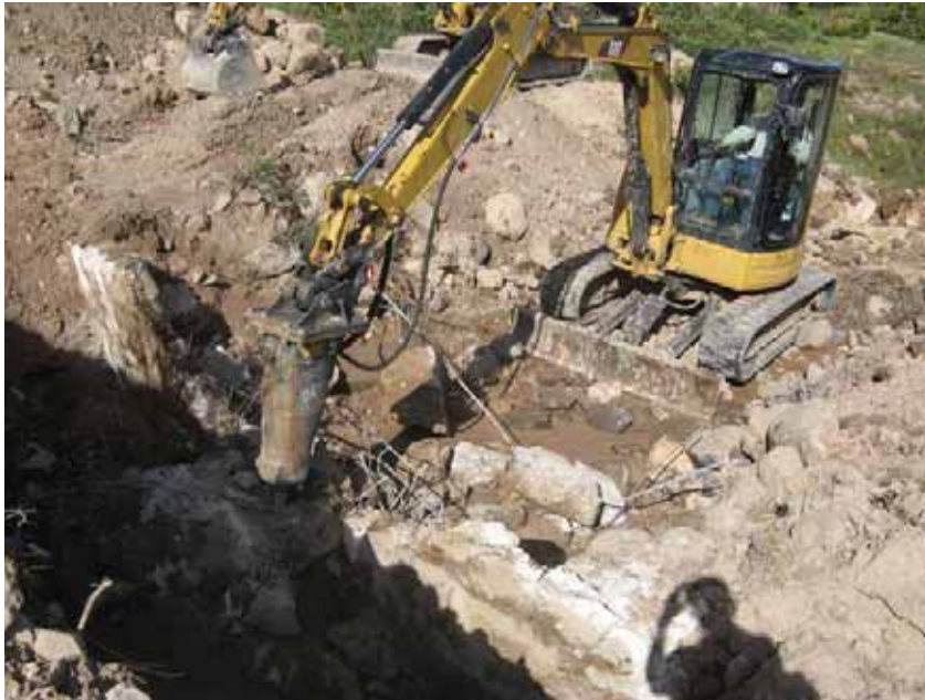
Figure 14: Inlet structure being removed using a stinger attachment.
