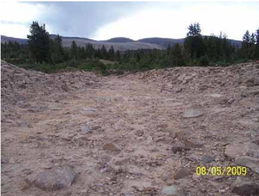
Figure 22: View of finished channel at Five Point from top gabion, looking downstream.
