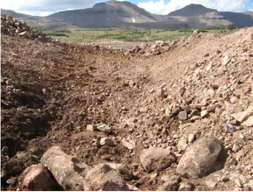
Figure 40: Completed breach prior to placing gabion cutoff walls and riprap.
