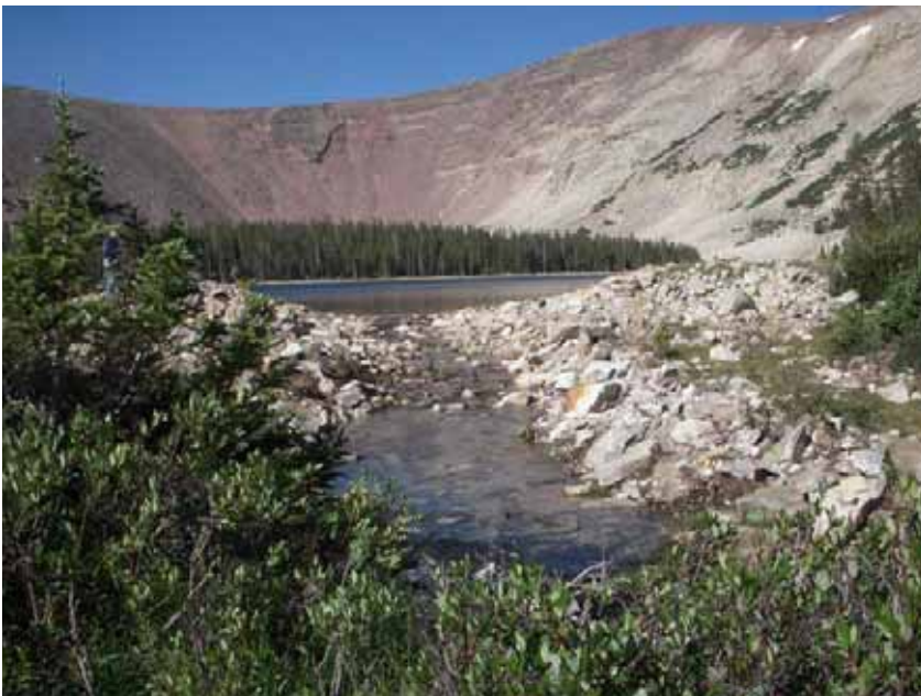
Figure 27: Looking upstream to the finished channel w/ riprap in place.
