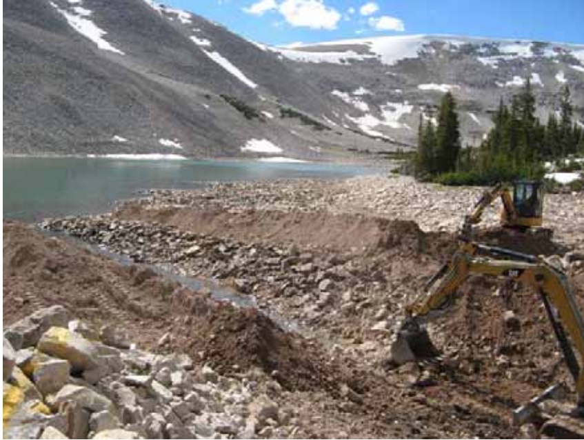
Figure 31: Crew cutting final grade.
