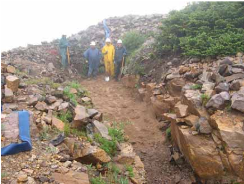
Figure 48: Sand filter in place at plugged outlet.
