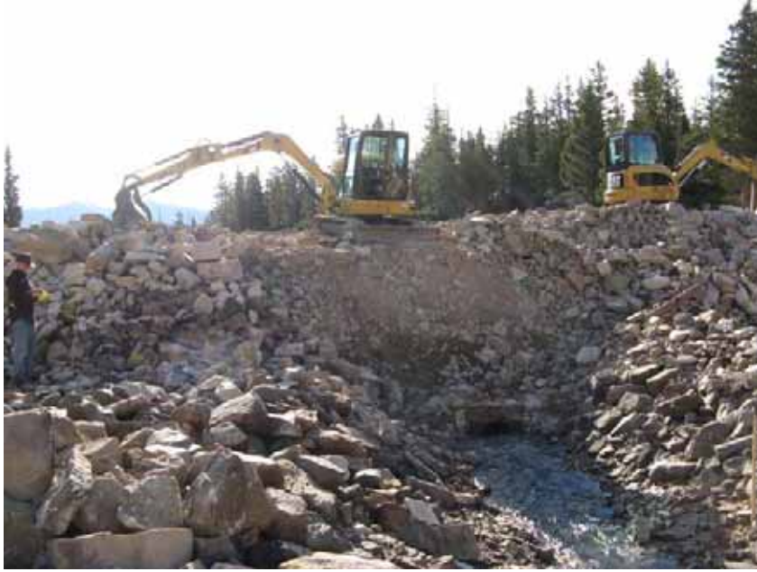
Figure 30: Crew working on removing riprap from existing channel.
