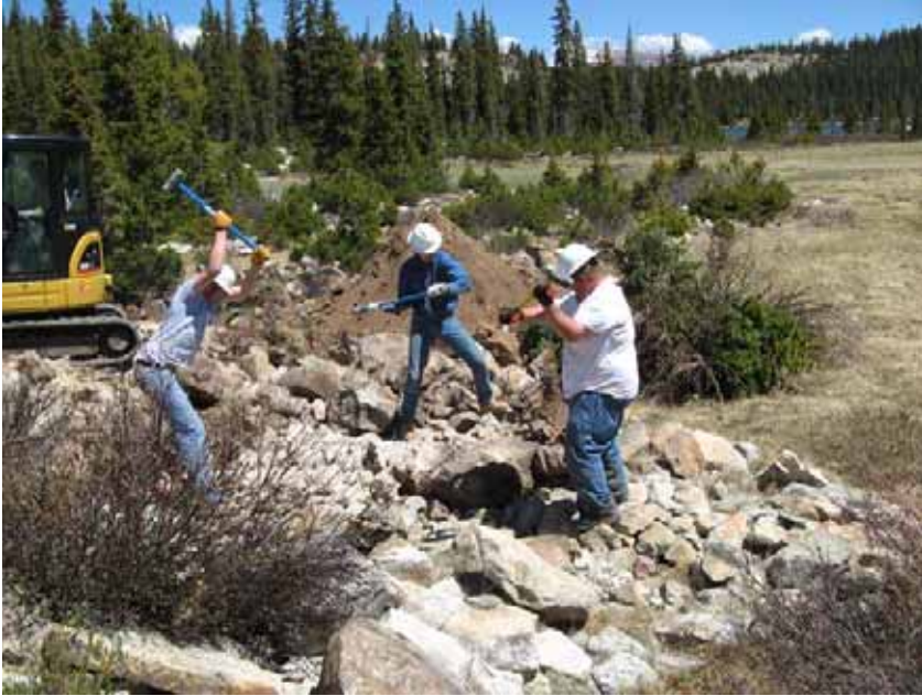
Figure 26: Hand crew assisting with breaking up concrete structure with sledge hammers which was proven ineffective, so they used the stinger attachment to get the job done. Bluebell Lake.
