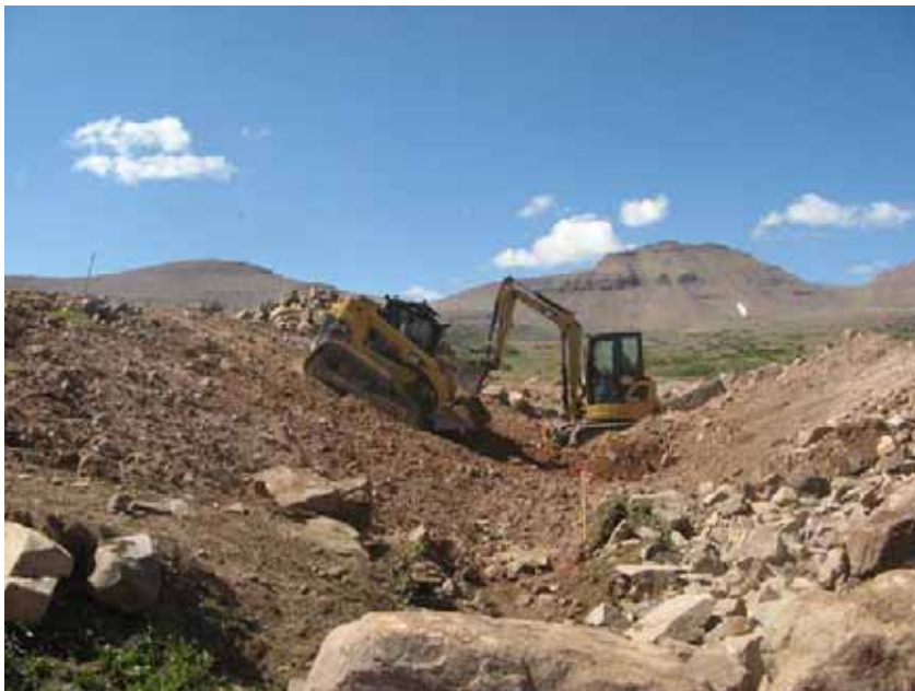
Figure 39: Crew cutting through dam at Superior Lake.
