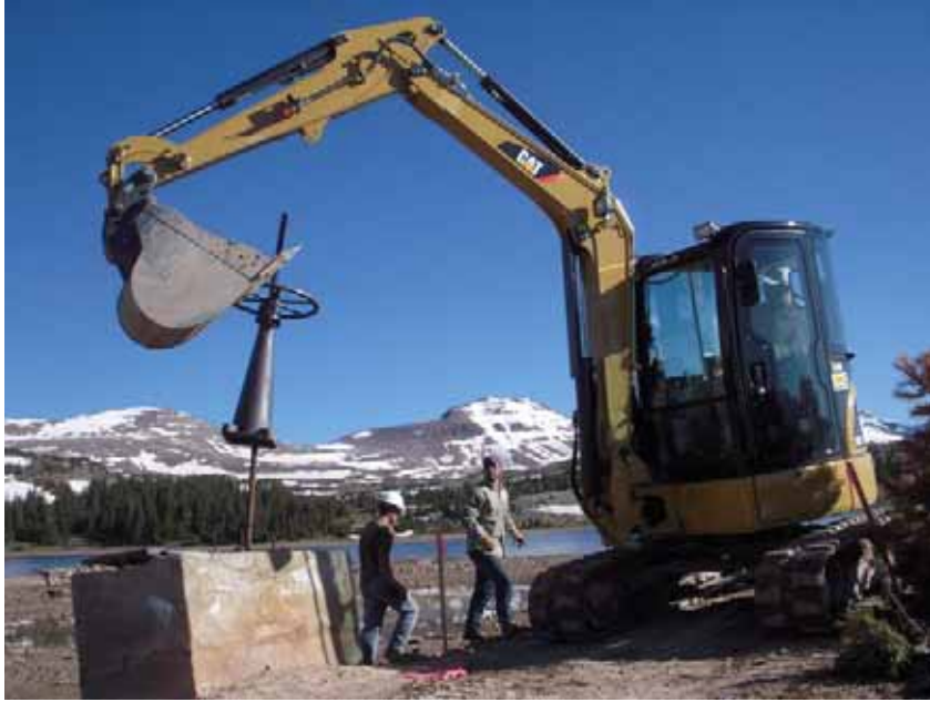
Figure 8: Crew using trackhoe to remove outlet works at Five Point.
