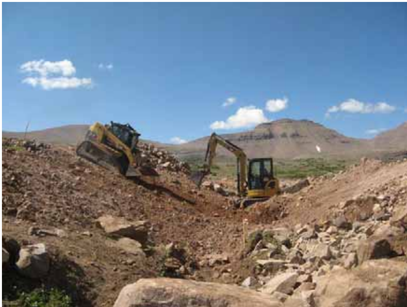
Figure 44: Placing riprap after cutoff walls were in place.
