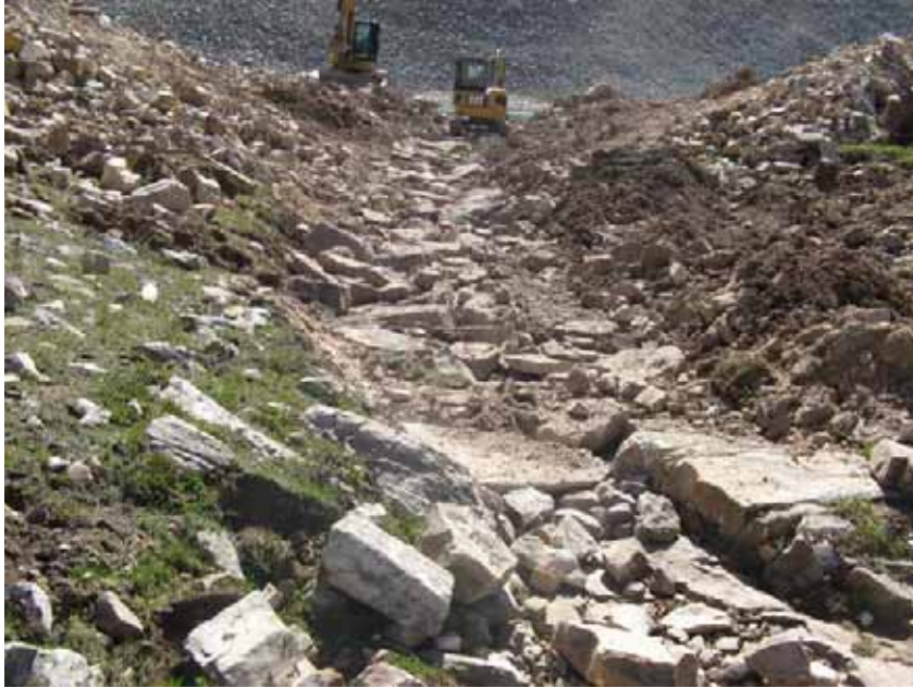
Figure 35: Rock sills in place.
