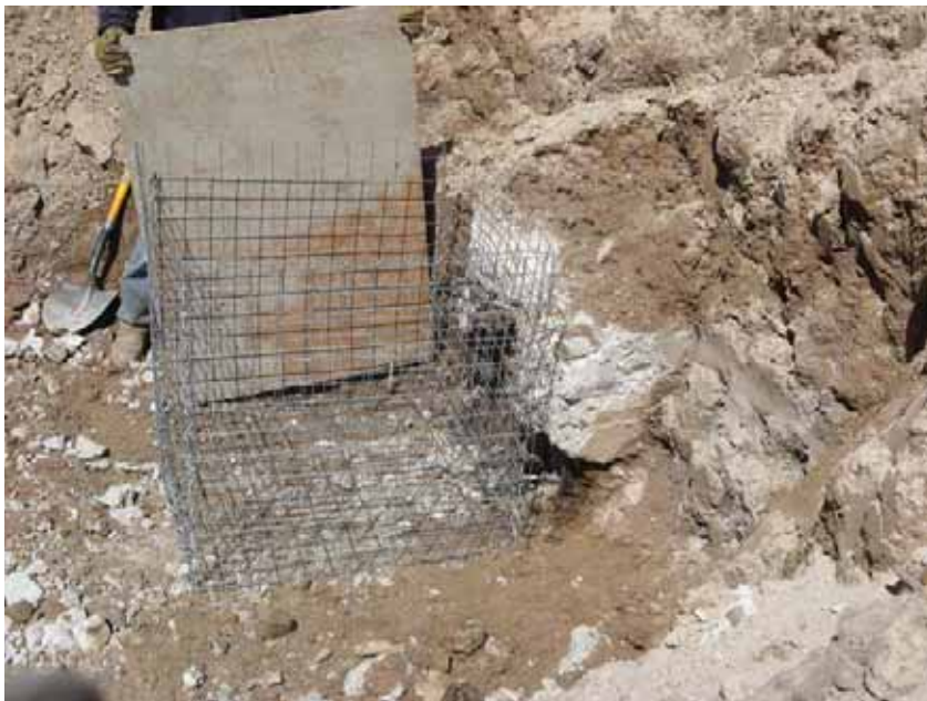
Figure 15: Installing gabion basket at outlet pipe prior to grouting.
