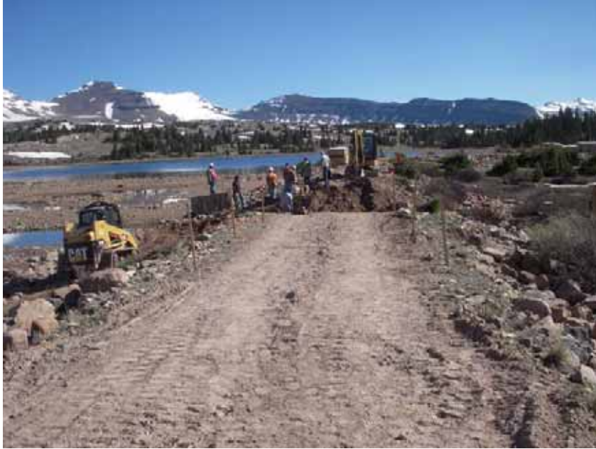
Figure 6: Crew cutting the breach through the Five Point dam.
