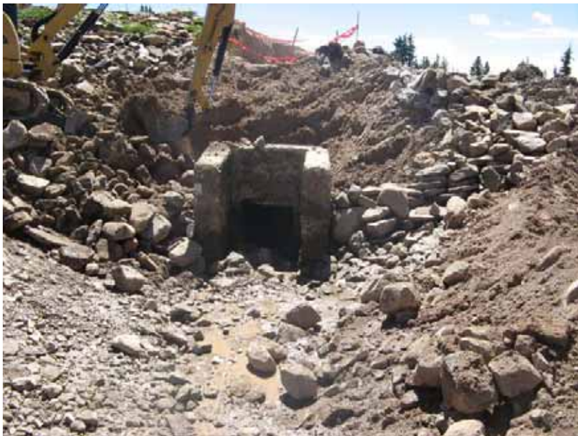
Figure 9: Removing inlet structure at Five Point.
