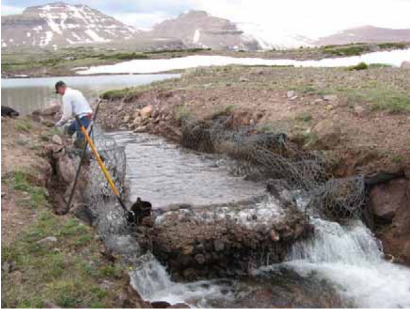
Figure 40: Hand crew removed gabions from old spillway.
