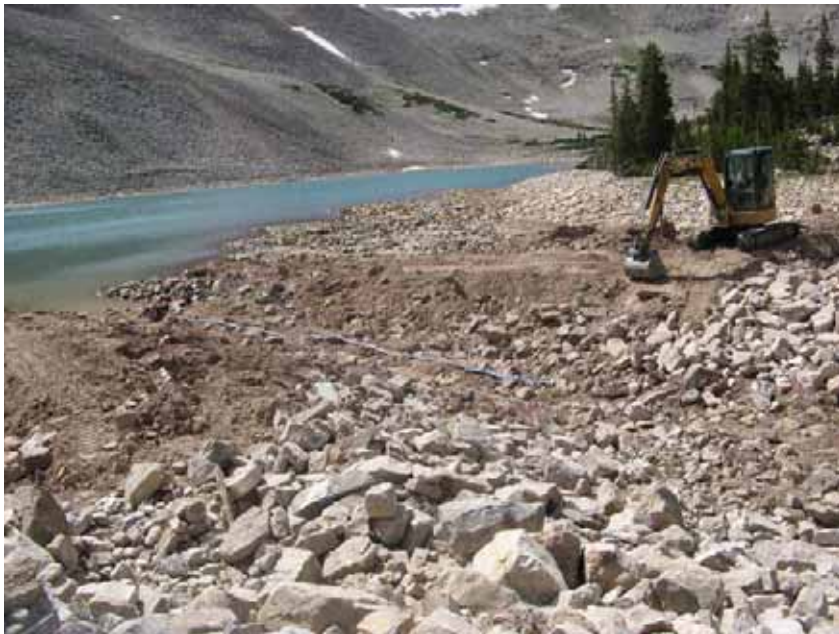
Figure 36: Crews continue to place riprap along the sides of the new outlet channel.
