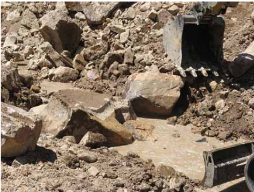
Figure 34: Rock sills placed in channel.
