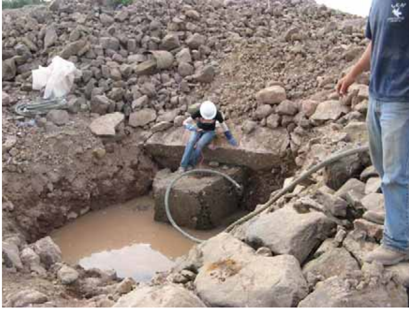
Figure 47: Crew sealed outlet pipe by placing 3'x3'x3' gabion basket filled with rock and grout on the upstream side of the outlet pipe.
