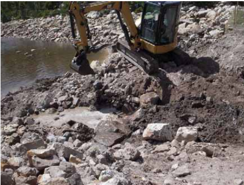
Figure 25: Crew installing rock sills at Bluebell Lake.
