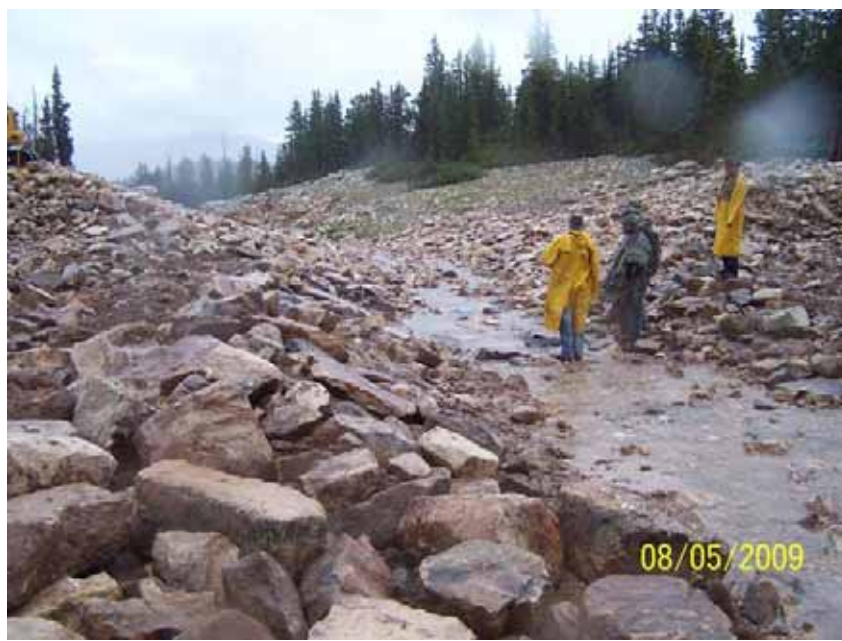
Figure 38: Looking downstream through the completed breach channel at Drift Lake.
