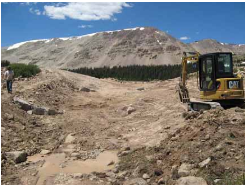
Figure 17: Breach channel prior to placing riprap.
