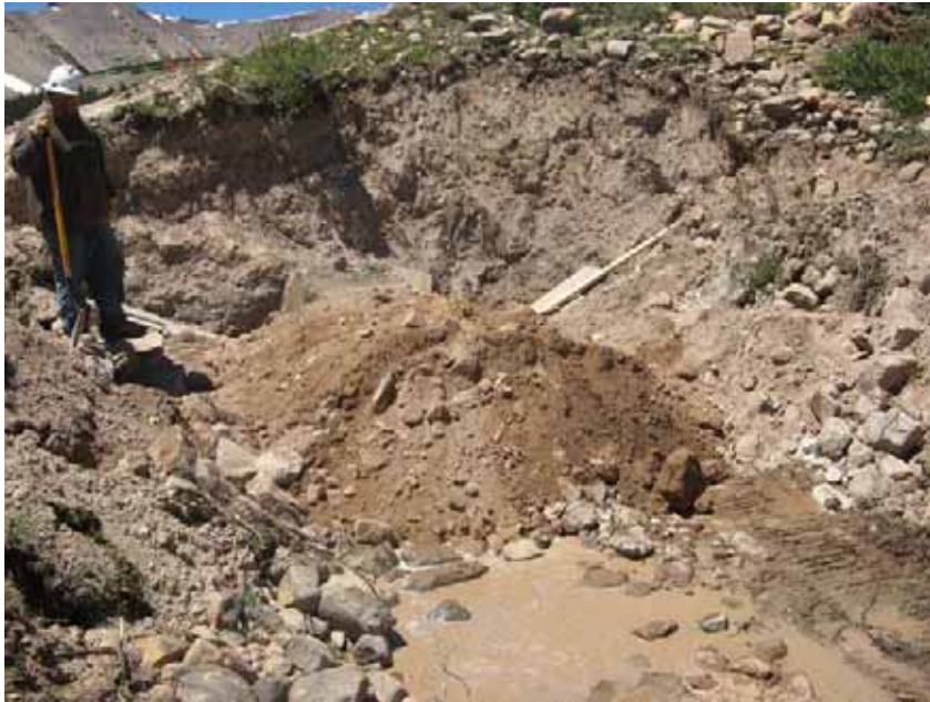
Figure 16: Grouted outlet pipe with sand filter in place.
