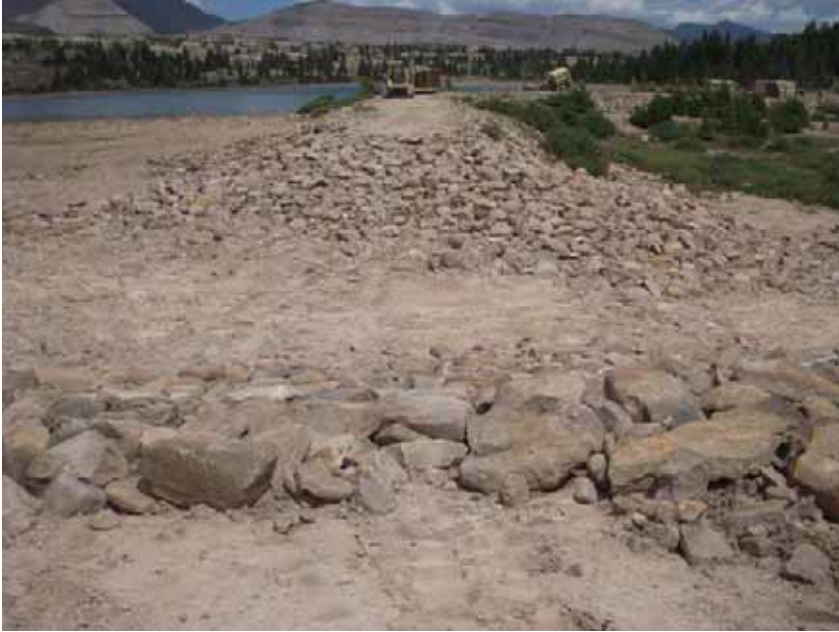
Figure 21: View of finished channel at Five Point graded and lined with riprap.
