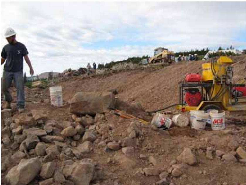
Figure 50: Grouting operation underway for plugging the outlet pipe.
