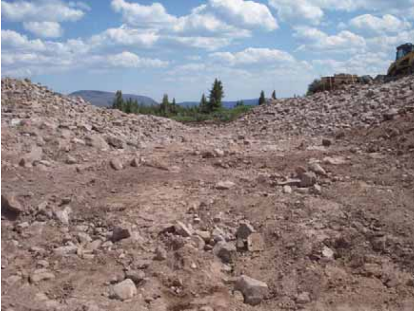
Figure 49: New breach at Superior Lake after work was completed.
