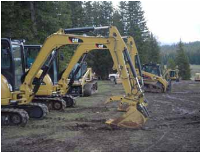
Figure 3: Equipment used at Garfield Basin.
