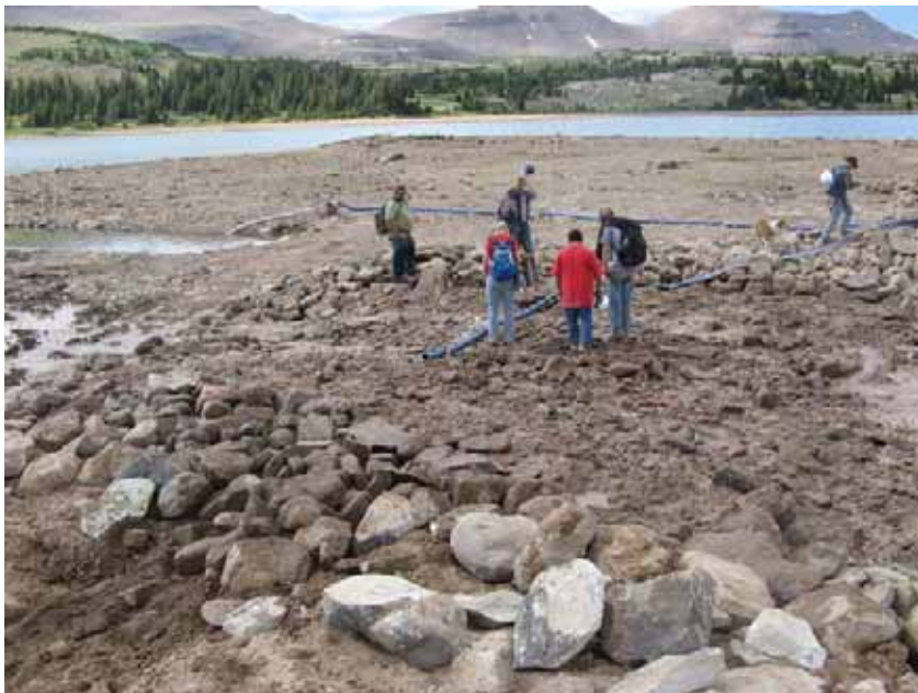
Figure 19: Hand crew washing fines into new outlet channel.
