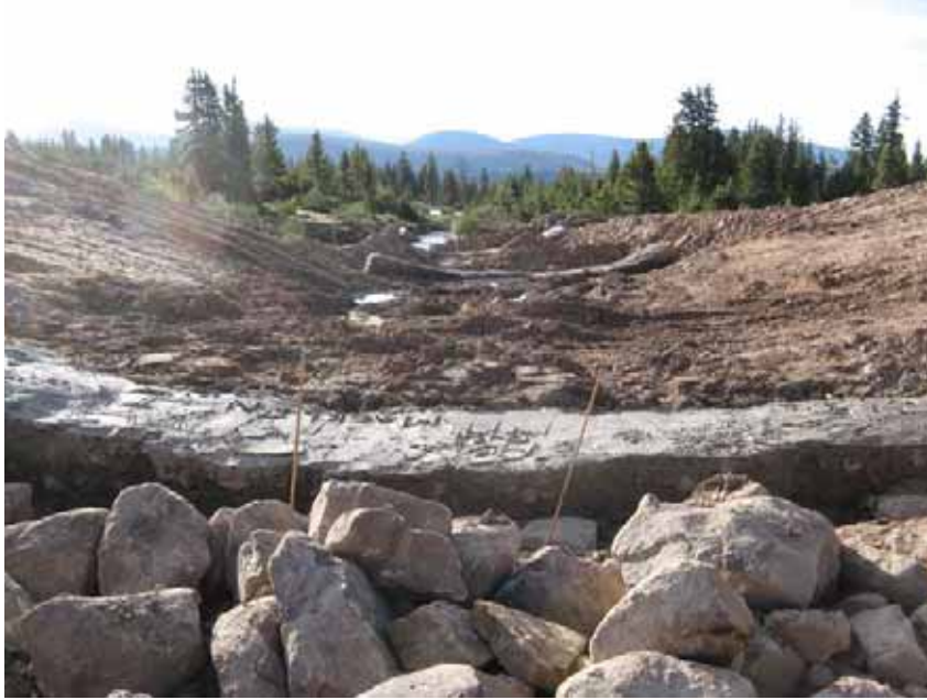
Figure 12: Five Point Lake Dam breach looking downstream with the gabion cutoff walls in place.
