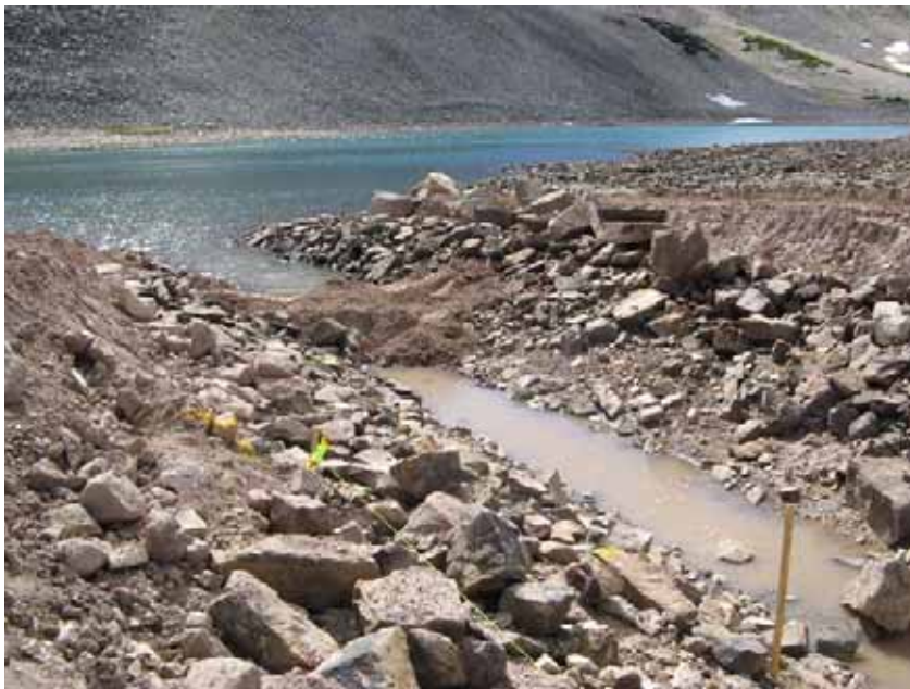
Figure 32: Temporary coffer dam put in place to control water flow.
