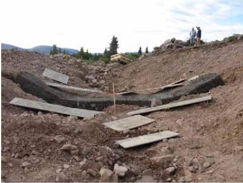
Figure 43: Grouted middle cutoff wall in place with forms removed.
