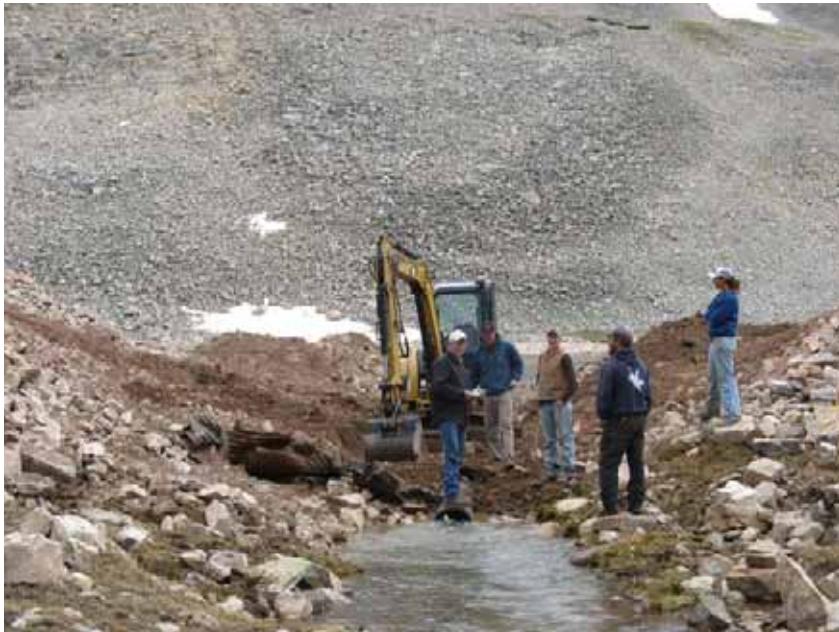
Figure 30: Crew cut through dam and removed the outlet pipe.
