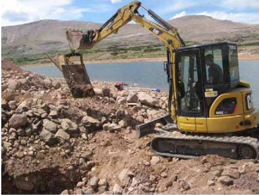
Figure 46: Removing the upstream portion of the outlet pipe.
