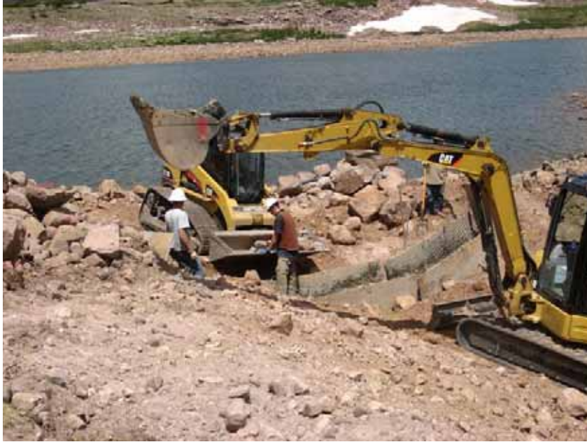
Figure 41: Placing of cutoff wall at top of breach.
