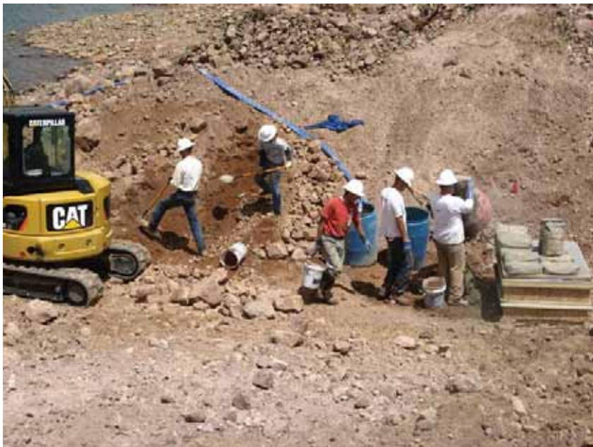
Figure 42: Grouting operation for the gabion cutoff walls.
