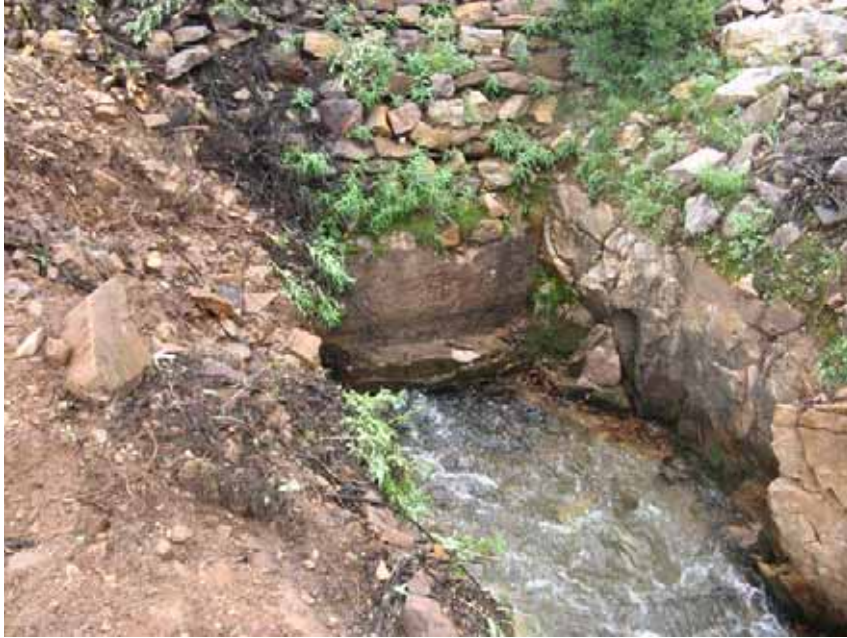
Figure 41: Outlet channel prior to construction.
