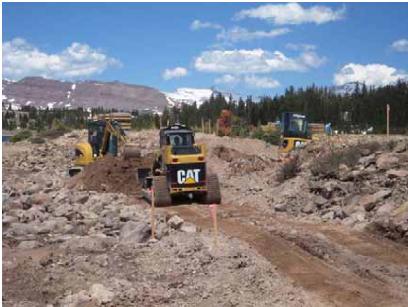
Figure 7: Skid Steer and trackhoe used to make the cut.
