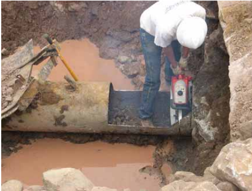
Figure 45: Hand crew cutting off a portion of the outlet pipe prior to grouting.
