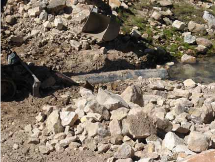
Figure 33: Crew used trackhoe to remove the outlet pipe.
