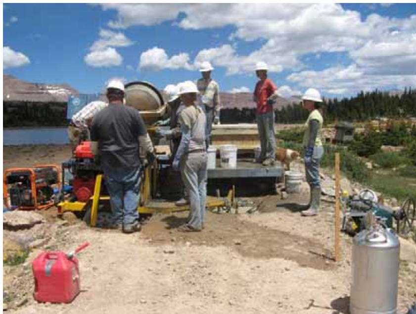
Figure 11: Grouting operation with DCWCD hand crew for cutoff walls.
