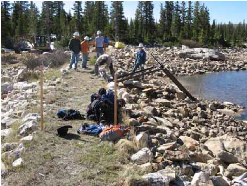
Figure 23: DCWCD crew removing headgate.
