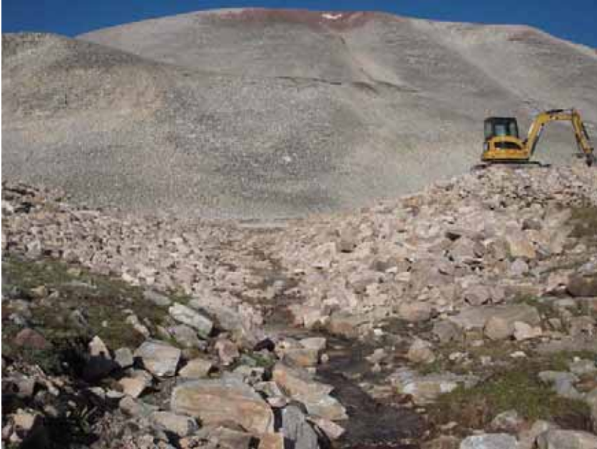
Figure 37: Looking upstream on the completed breach channel at Drift Lake.
