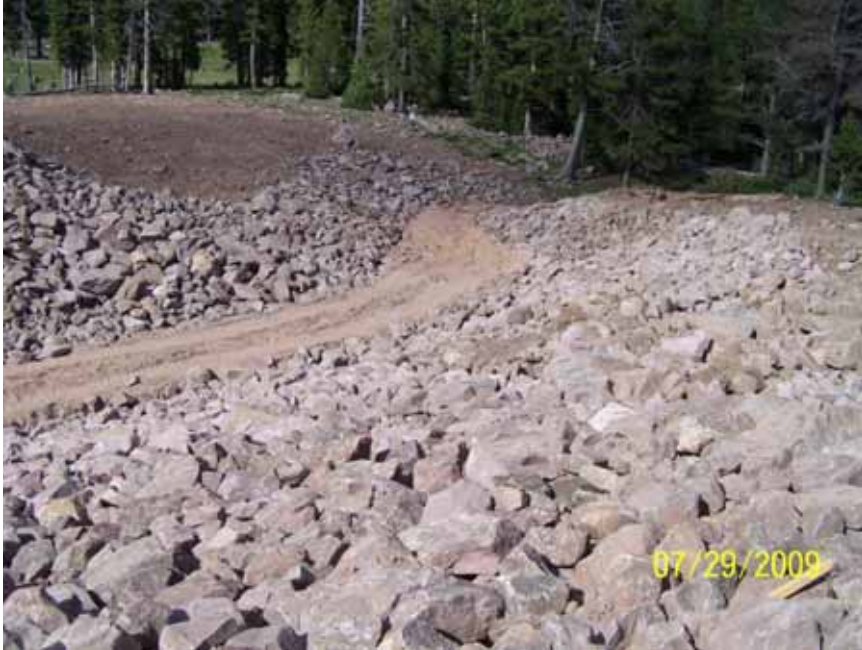
Figure 16: Looking downstream to the completed breach channel at Kidney Lake.
