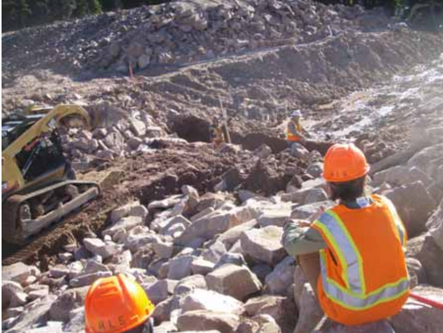
Figure 9: Installation of the second cut-off wall.
