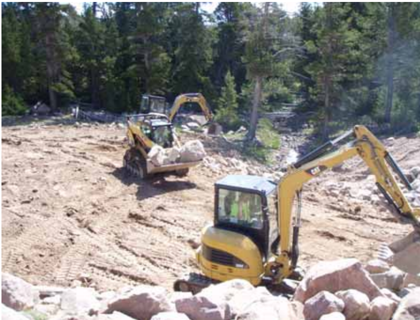
Figure 11: Reclamation crew placing riprap in the channel.
