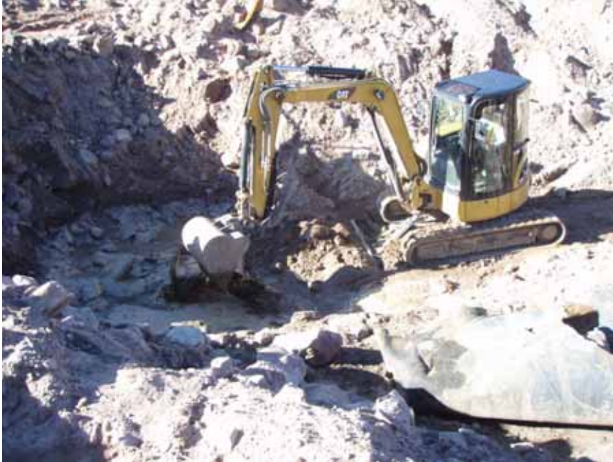
Figure 13: Demolition of inlet structure using trackhoe.
