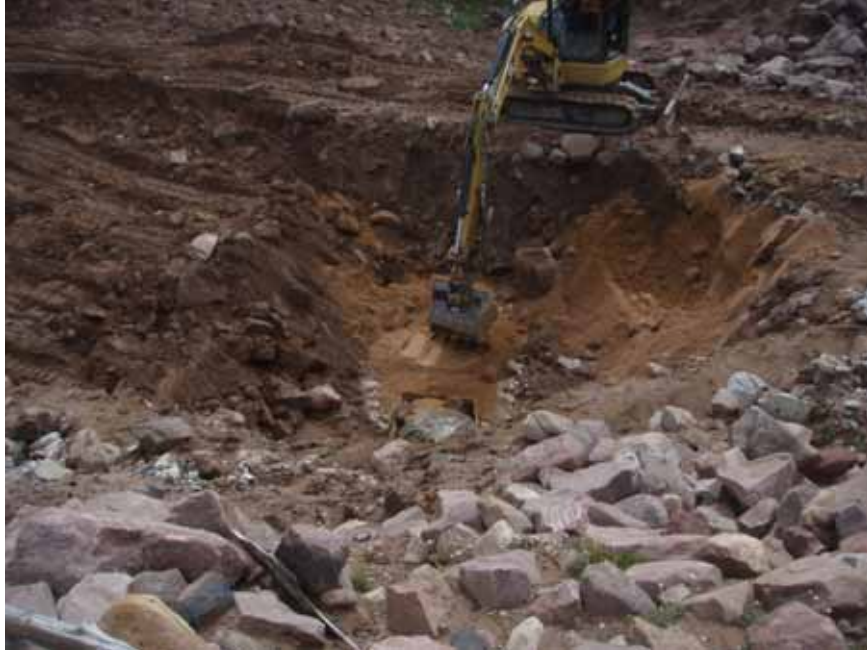
Figure 15: Grouted outlet pipe with sand filter at downstream end.
