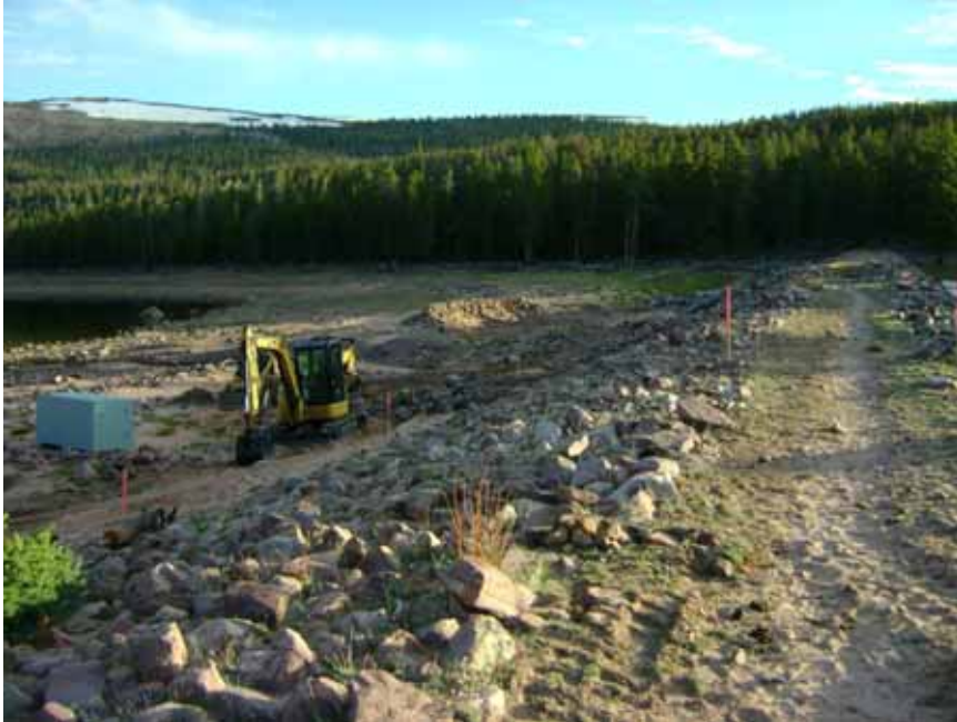
Figure 4: Reclamation crew working on removing riprap.
