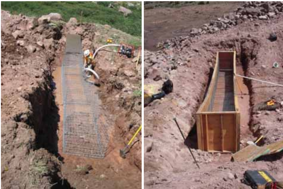
Figure 12: Gabion cutoff walls with forms and #9 wires ((3) 3'x4'x9').
