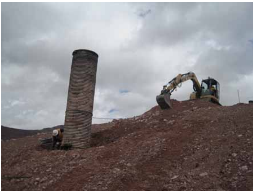
Figure 19: Randy Crozier cutting the 48 inch gate well tower with a torch.
