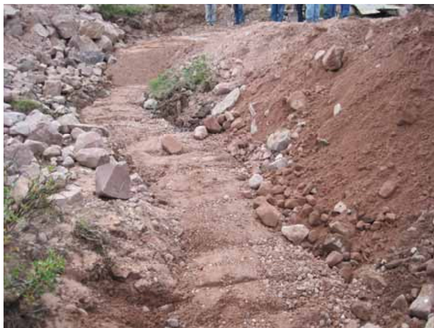
Figure 25: Looking upstream to sand filter and pea gravel drain in place on downstream side of outlet pipe.
