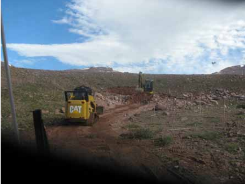
Figure 4: Crew using trackhoes and skidsteers to excavate breach.
