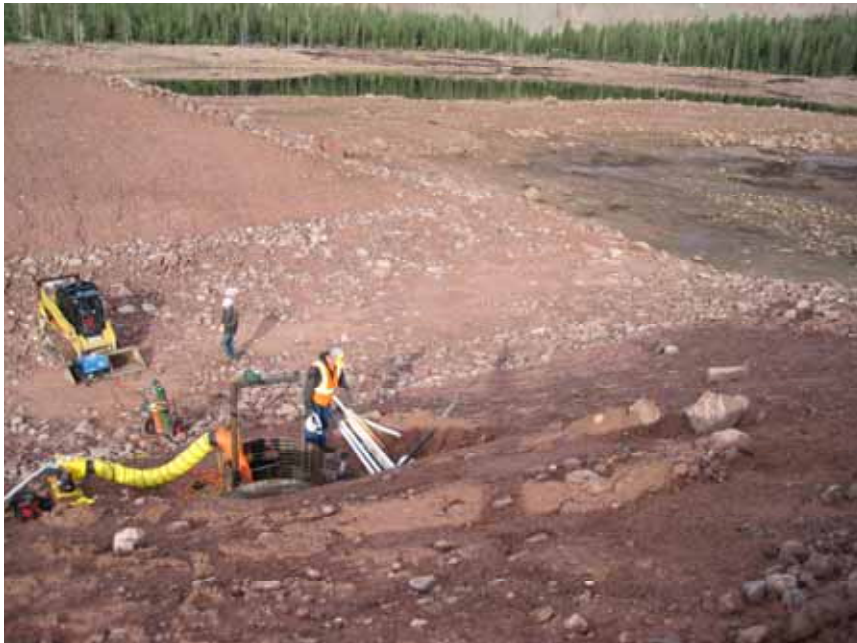
Figure 20: Crew preparing for confined space entrance into gate well.
