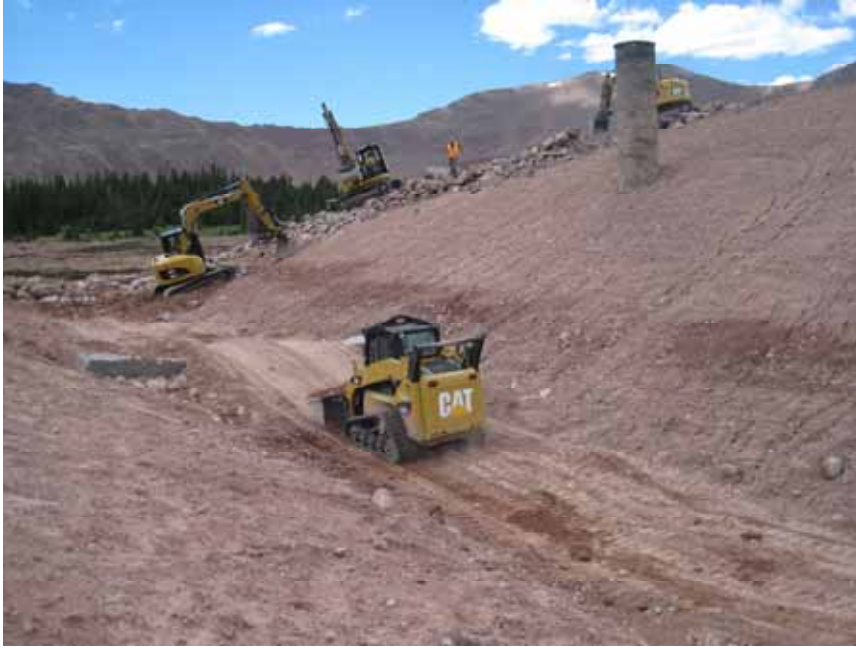
Figure 18: Skidsteer transporting rip-rap and fines while trackhoes place riprap on breach.
