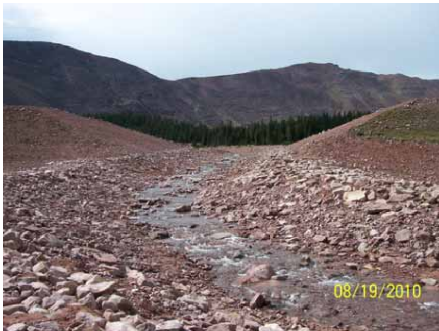
Figure 26: Looking upstream to the completed breach with water flowing through it.
