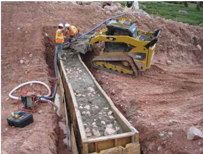
Figure 15: Crew pouring 3 rd gabion basket using skidsteer for transporting cement.
