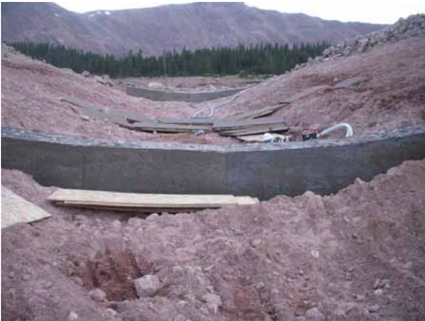
Figure 14: First and second gabion cutoff walls poured in place (looking upstream).
