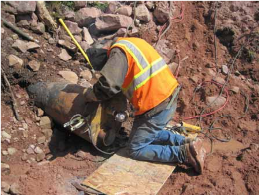
Figure 22: Randy Crozier welding steel plate on downstream end of pipe.
