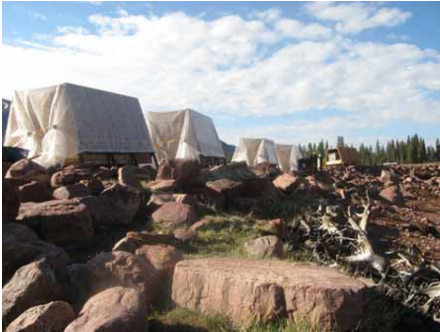
Figure 3: Fuel containment cover in place in preparation for blast.
