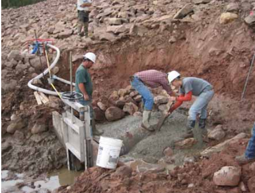
Figure 10: Crew batching and pouring cement on new head structure on existing outlet pipe.
