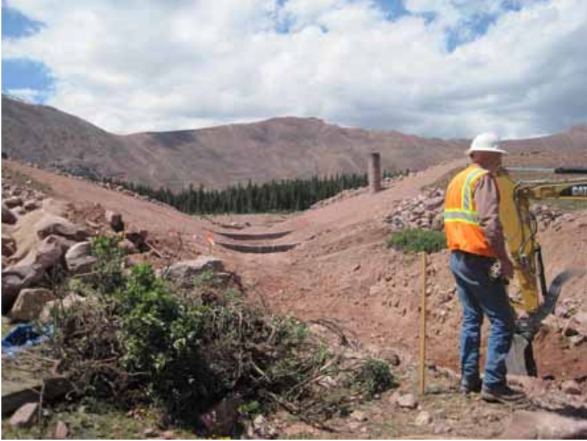
Figure 16: Looking upstream with three gabion walls in place.
