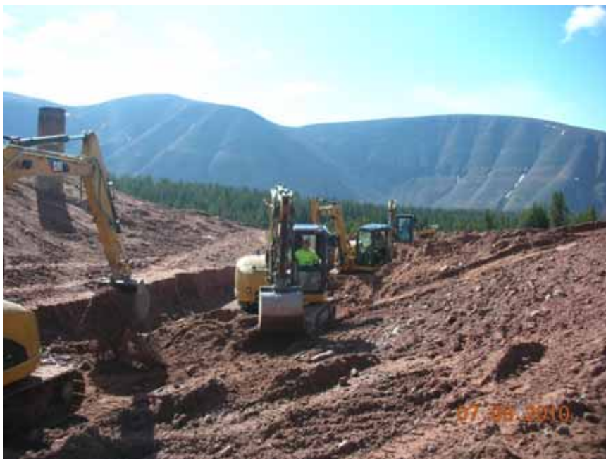
Figure 8: View of all four trackhoes working in breach before placing cut-off walls and riprap.
