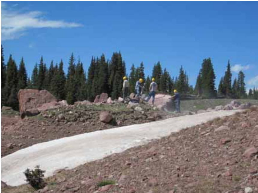
Figure 6: Forest Service blasters drilling and setting charge holes for blasting.
