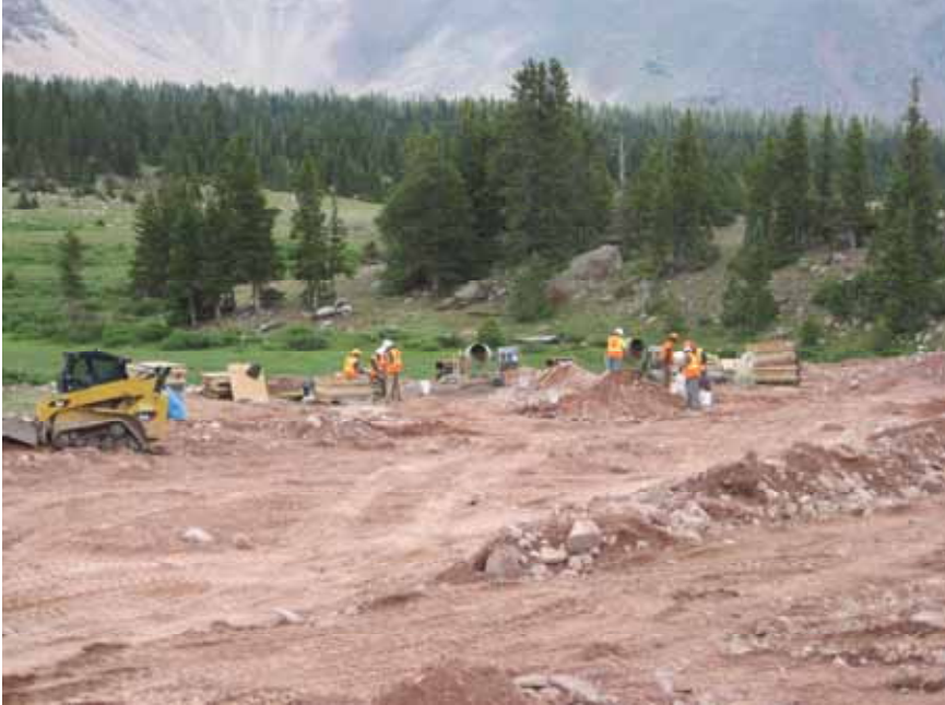
Figure 13: Crew mixing and delivering cement for gabion cutoff walls.
