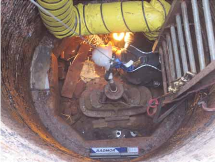
Figure 21: Randy Crozier in gate well welding in 1-1/4" nipples.
