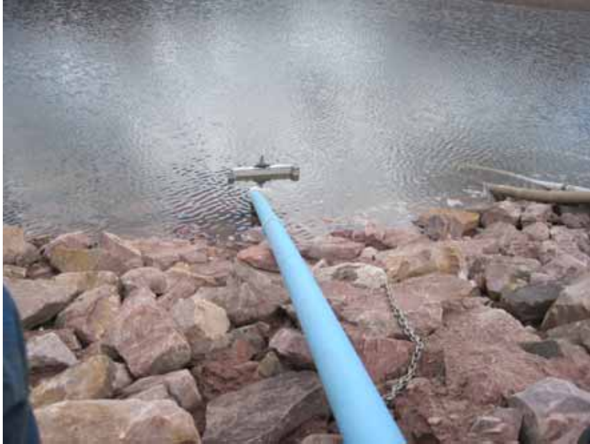
Figure 23: 4" vent pipe on upstream structure used for grouting; it was broken off when grouting operation was completed.
