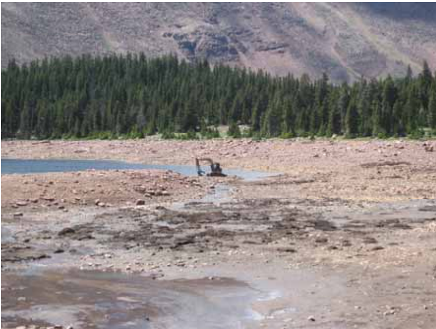
Figure 17: Trackhoe excavating the lake connection channel.
