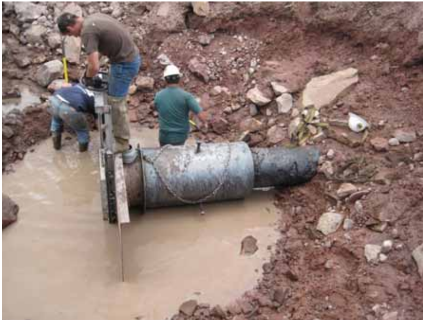
Figure 9: DCWCD and UCC crews installing head structure (designed for up to 30lb back pressure).
