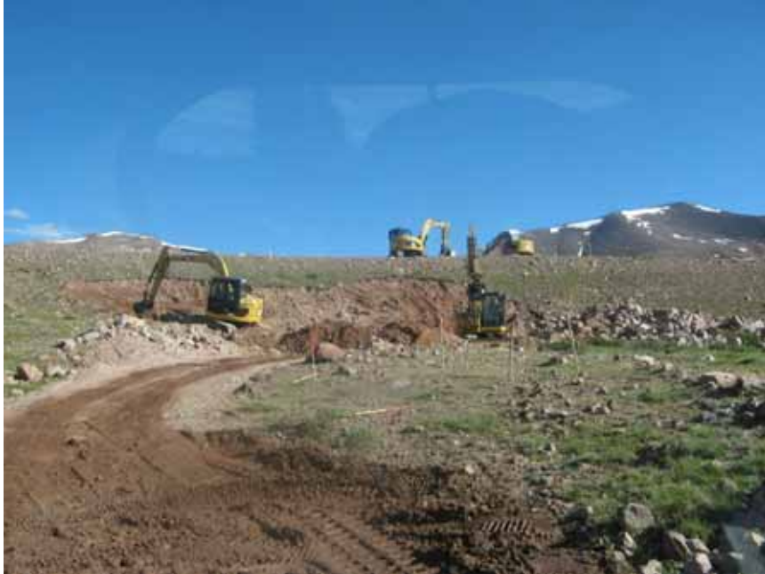
Figure 7: Four trackhoes were used to excavate the breach while six skidsteers hauled the material to the spoil pile.
