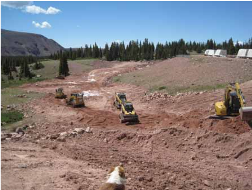
Figure 5: Material was removed from the dam and transported to spoil areas in an assembly line fashion.
