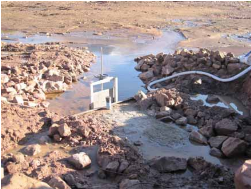
Figure 11: View of new head structure with concrete poured around existing outlet pipe.
