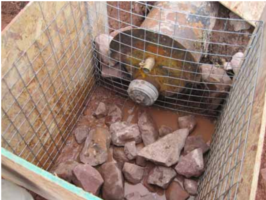
Figure 24: 3'x3'x3' gabion at downstream end of pipe.
