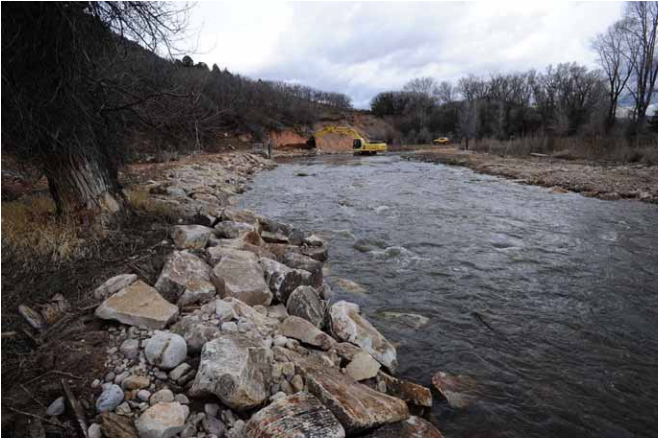
Figure 11. Photograph of the newly-constructed bank and rock protection downstream of the new structure. This photo also shows the constructed riffle at a somewhat higher discharge than is shown in Figure 10.
