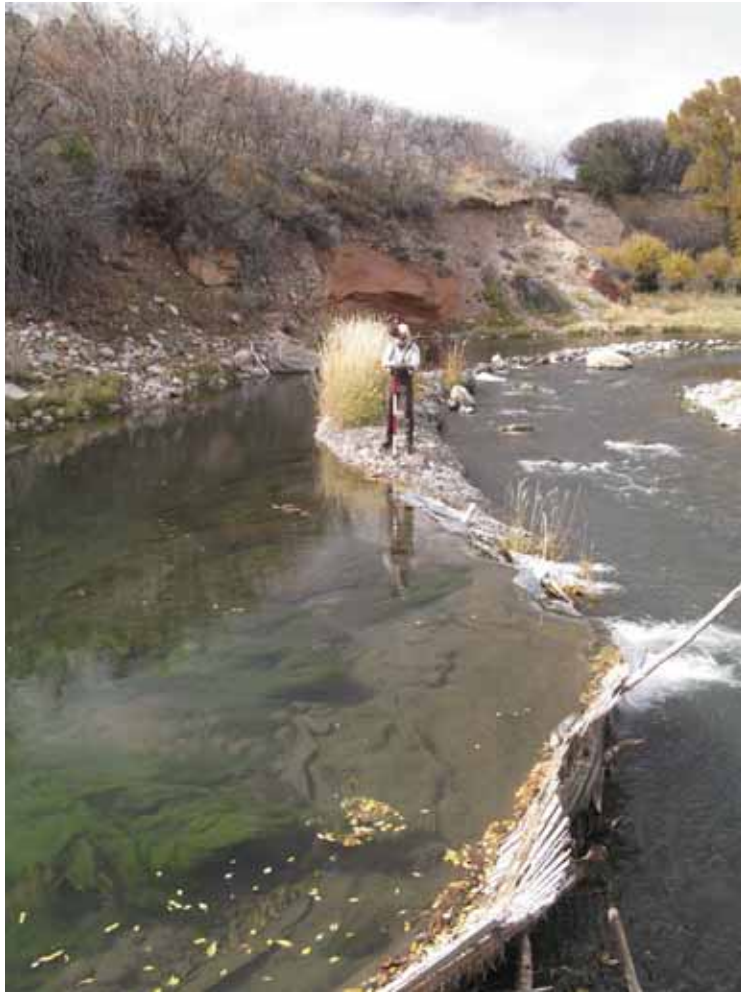
Figure 6. Photograph of the pre-project sill at the Turnbow Diversion, showing miscellaneous debris used in the sill.
