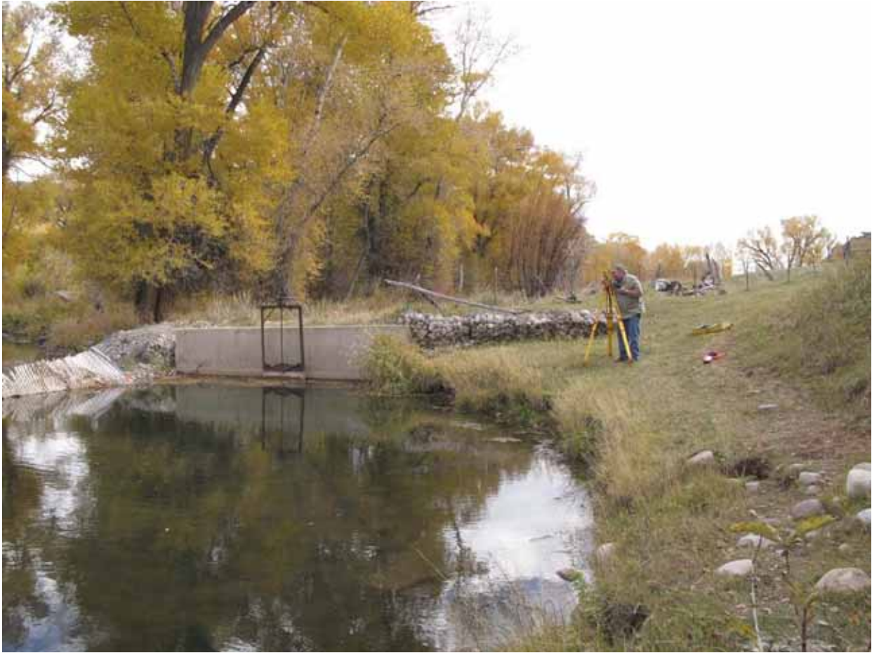
Figure 7. Photograph of the pre-project headwall and gabions at the Turnbow Diversion.
