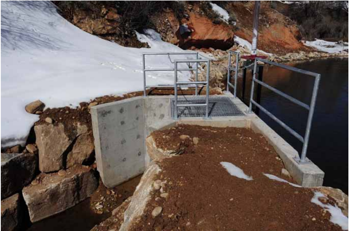
Figure 15. Photograph of the completed concrete diversion; with railings, gate, and grating installed.
