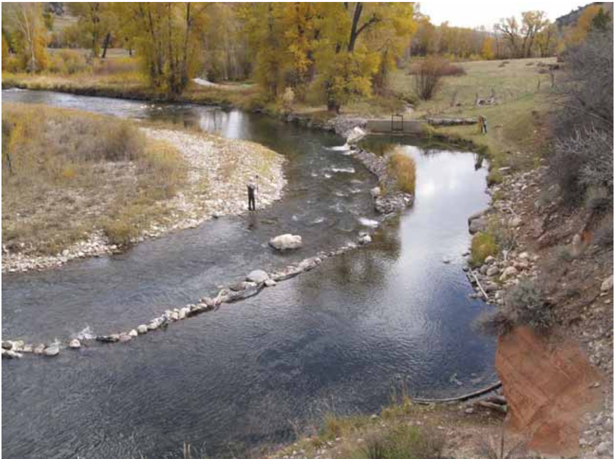
Figure 4. Photograph of the pre-project sill and headwall at the Turnbow Diversion, taken from cliffs on river right, looking downstream.
