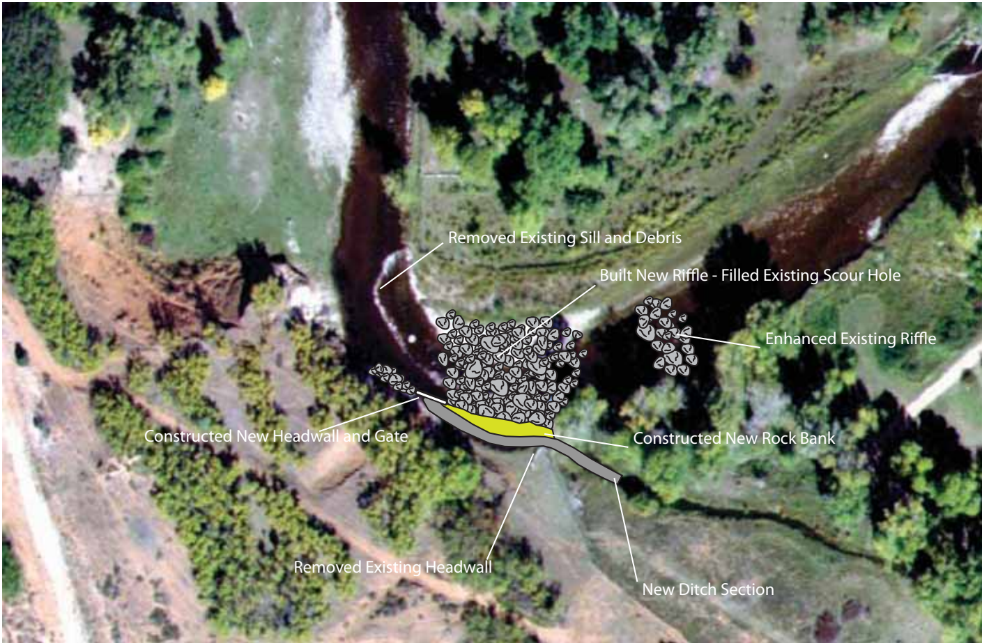
Figure 9. Completed action elements to rebuild the Turnbow Diversion.
