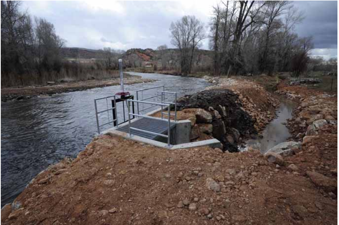
Figure 12. Photograph of the diversion area following construction: showing the concrete structure, the bank that divides the river channel from the new section of ditch, and the new riffle.
