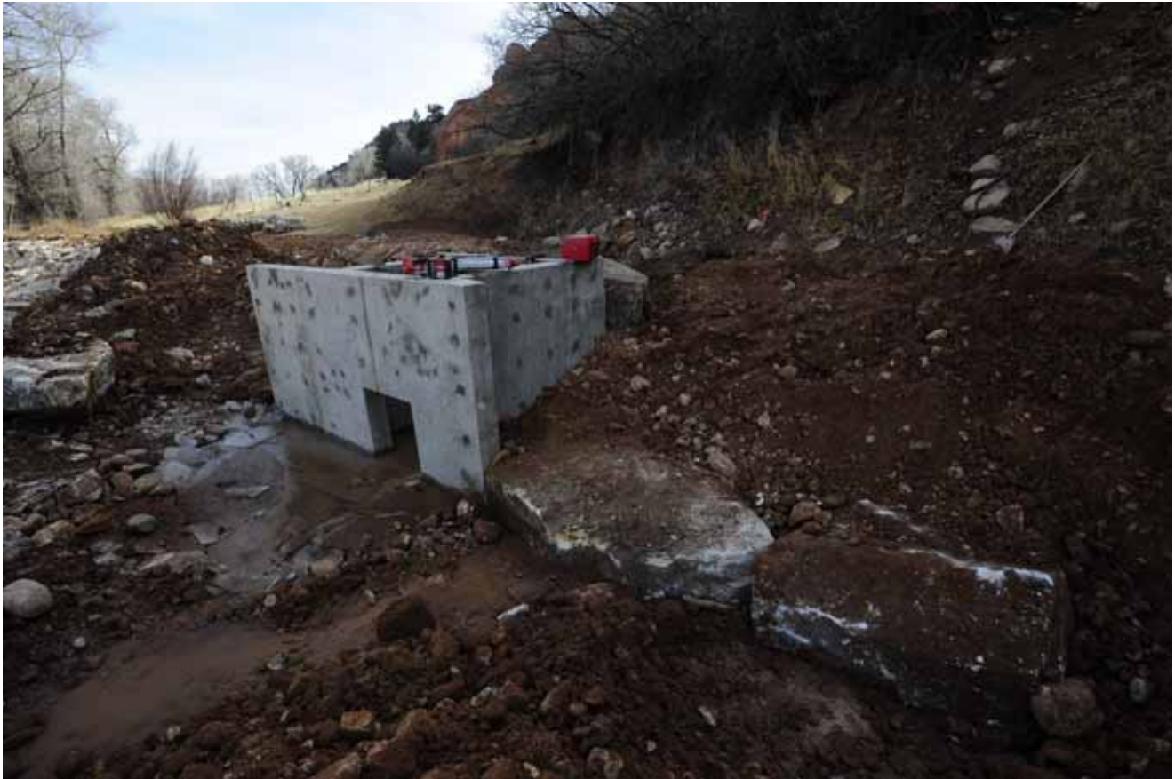
Figure 14. Photograph of the new diversion, during bank construction, showing large rocks that were placed to transition between the structure and new banks. The soil behind the large rock was compacted to limit seepage, using a trackhoe and a rolling compactor.
