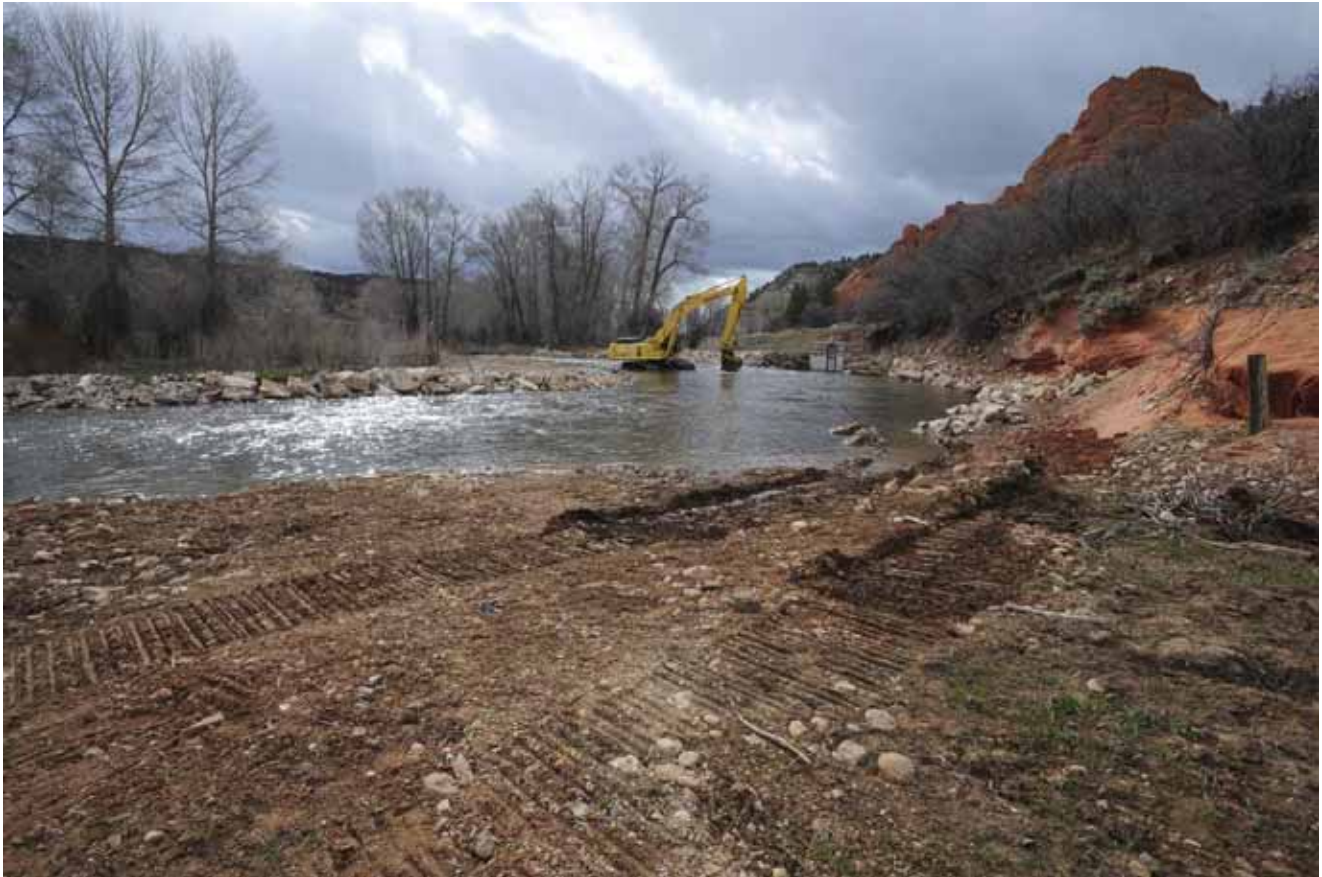
Figure 13. Photograph of the area immediately upstream of the new diversion. The new channel blends smoothly into the existing channel. Track marks from equipment were subsequently removed and the area was scarified and reseeded. The image was taken from river right, looking downstream.
