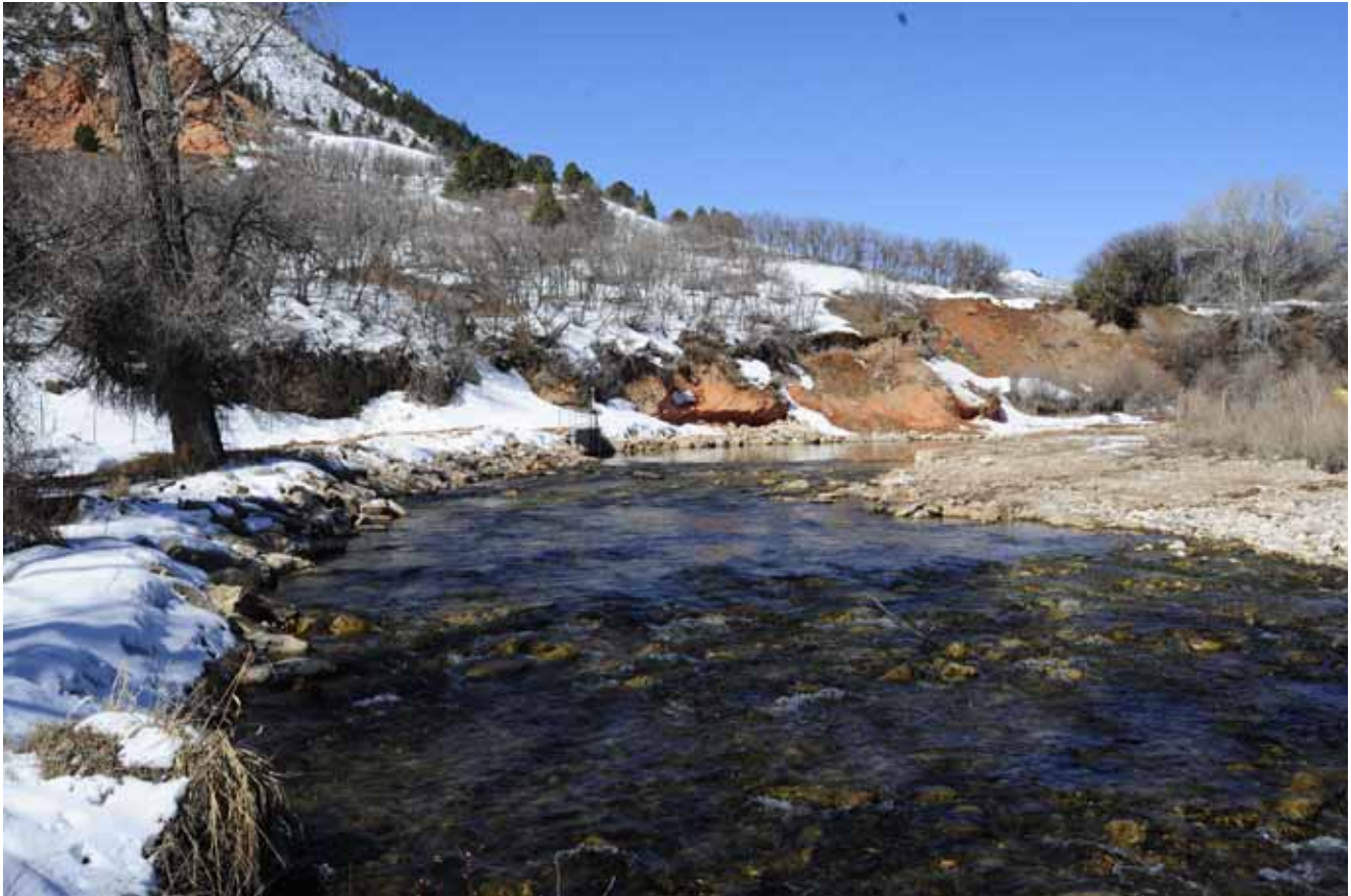
Figure 10. Photograph of newly-constructed riffle below the Turnbow Diversion. The riffle was constructed to have a natural form that does not promote erosion near the structure, and allows fish movement. This image was taken looking upstream. The new structure is visible near the center of the photo.
